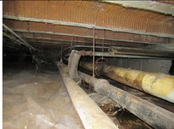
Photograph #2: View inside the crawlspace area below the hallway, near Room 106.
