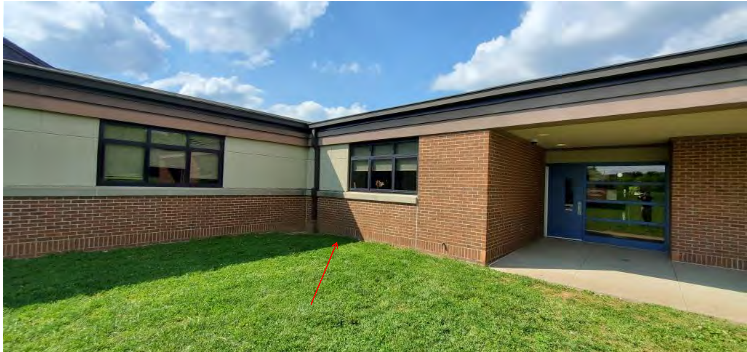
Figure 2: Outside view of Room #106.
