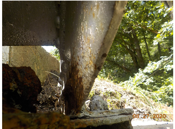
Abutment 2, right exterior gusset plate
