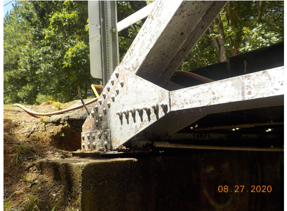
Abutment 2, left exterior gusset plate
