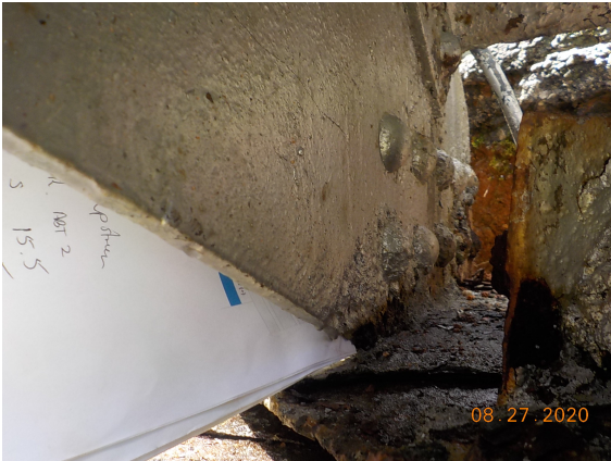
Abutment 2, left exterior gusset plate
