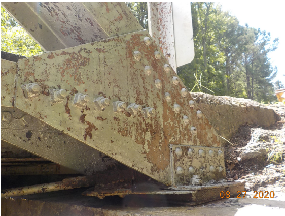
Abutment 2, right exterior gusset plate
