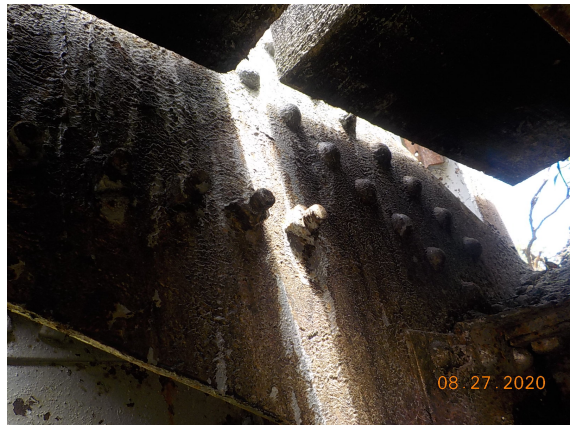
Abutment 1, right interior gusset plate.
