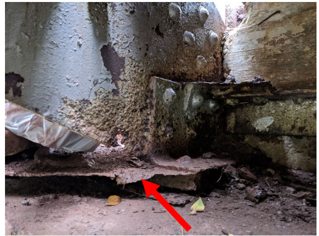
Base Plates and Bearing Pads
