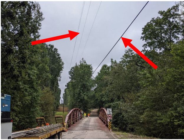
Jenkinsburg Road Bridge (Note Overhead Utilities)
