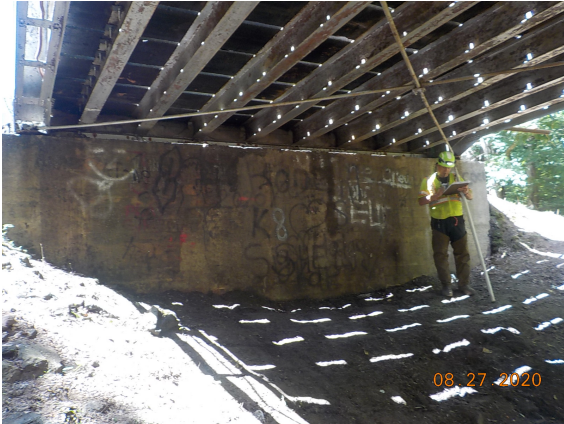
Looking at Abutment 2
