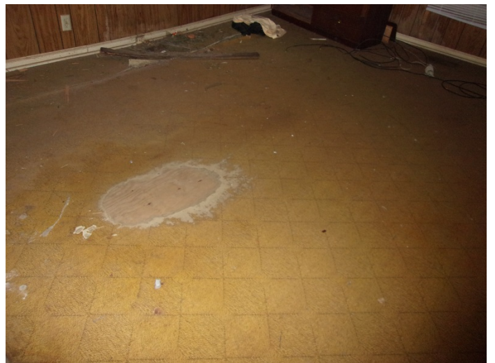
Photo 10 – Thatch pattern vinyl flooring with mastic in the bedroom.
