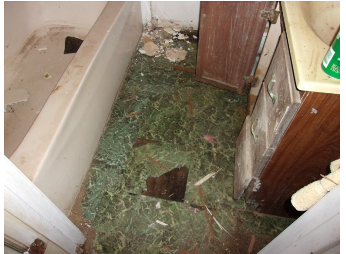
Photo 8 – 12" x 12" grey self-stick vinyl floor tile in the bathroom.
