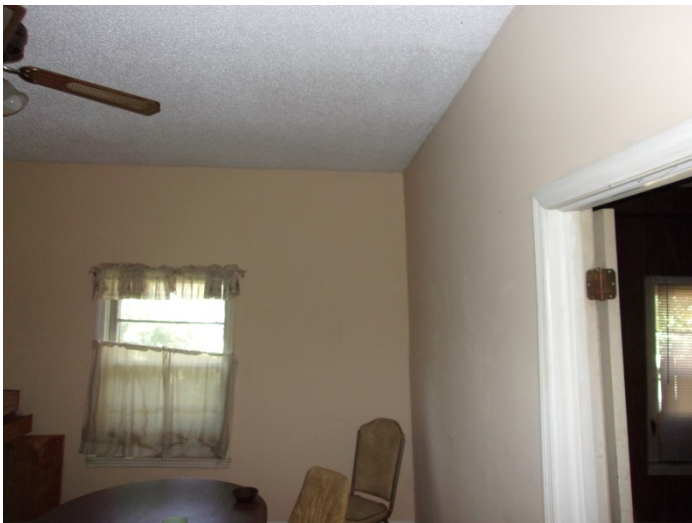
Photo 3 – Drywall with joint compound & tape throughout.
