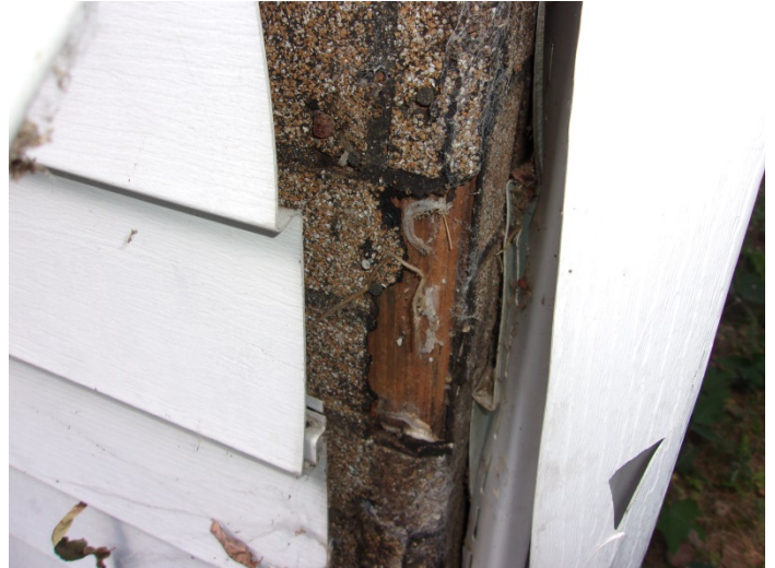
Photo 14 – Asphalt shingle siding under vinyl siding on the house.
