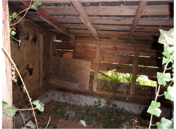
Photo 14 – Inside the exterior shed.
