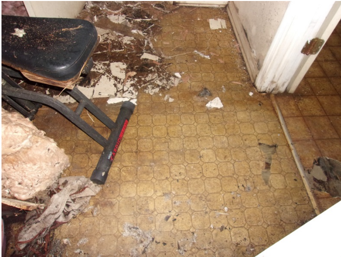
Photo 7 – Brown square pattern vinyl flooring with mastic in the hallway.
