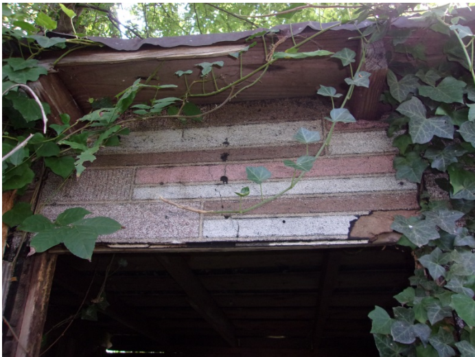
Photo 13 – Asphalt shingle siding on the exterior shed.
