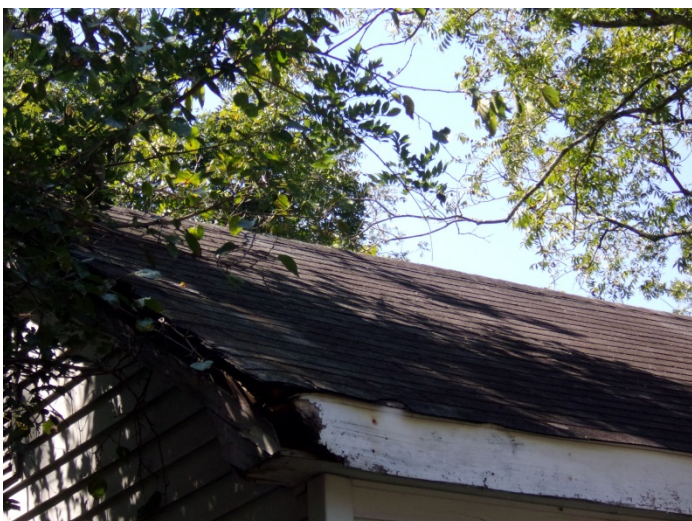
Photo 11 – Roof shingles & felt on the house roof.
