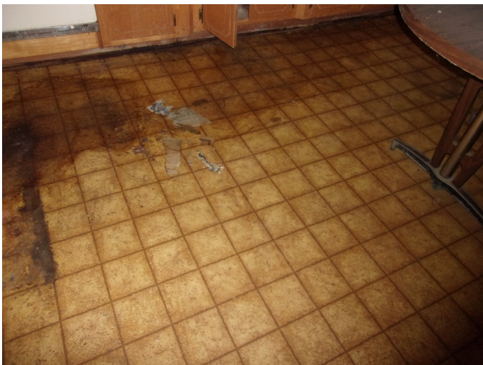
Photo 9 – Yellow large square pattern vinyl flooring with mastic in the kitchen.
