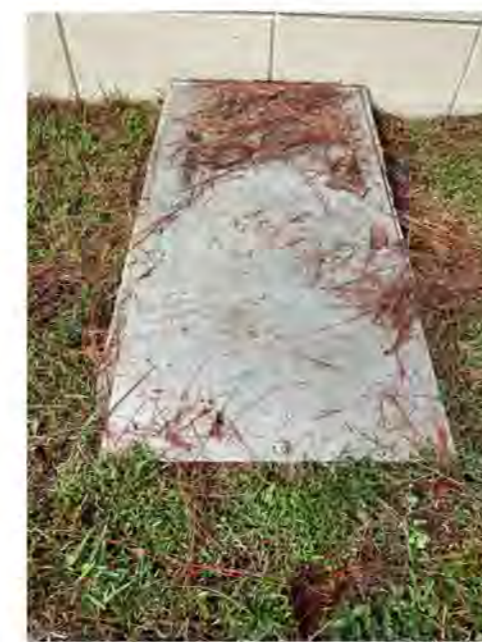
Photo No. 3 Concrete Utility Vault
