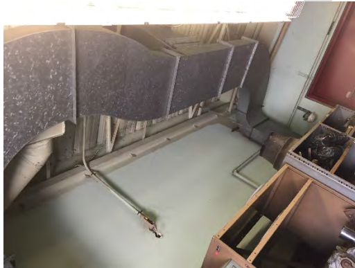
Ventilation and ductwork at corrosion room
