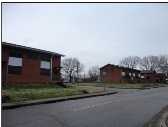
Austin Homes Apartments to the west along S Bell Street.
