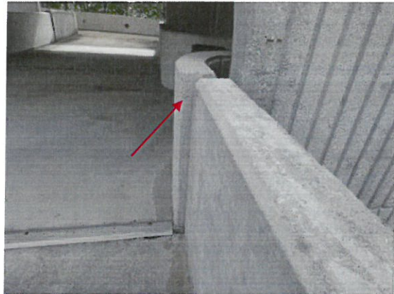
Photo 14: Horizontal differential displacement between parking structure C and stair tower
