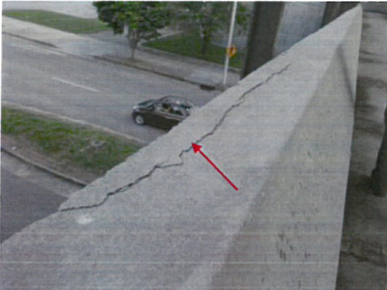
Photo 33: Concrete delamination on top exterior edge of edge beam on pedestrian bridge
