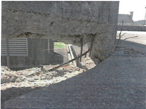
Photo 39: Deterioration of retaining wall on Parking Structure B
