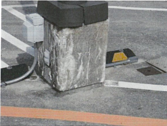
Photo 13: Deterioration of concrete pedestal
