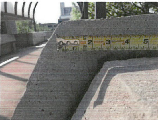
Photo 29: Horizontal differential movement between both sides of expansion joint on pedestrian bridge
