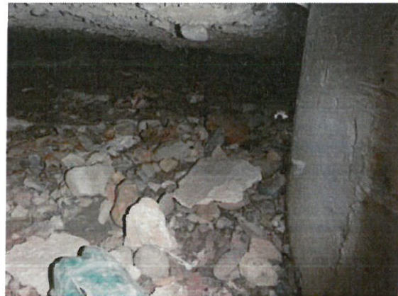
Photo 40: Voids underneath entry ramp on top level of Parking Structure B
