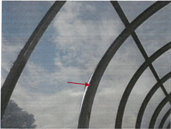
Photo 37: Detached canopy panel on pedestrian bridge
