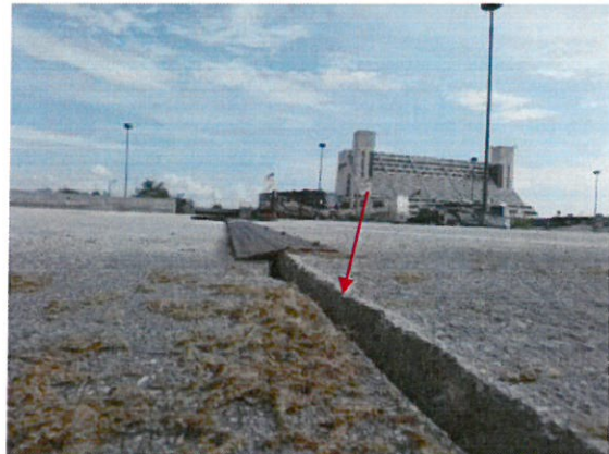
Photo 16: Differential vertical elevation on slab along expansion joint on roof level
