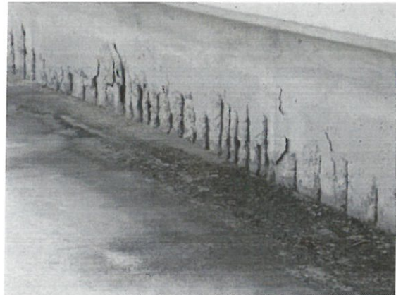
Photo 32: Concrete spalls on interior face of edge beam on pedestrian bridge
