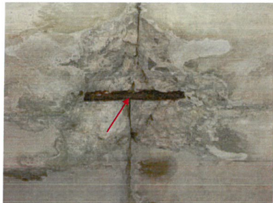
Photo 10: Close-up of concrete spall in joist (notice section loss in reinforcing steel)
