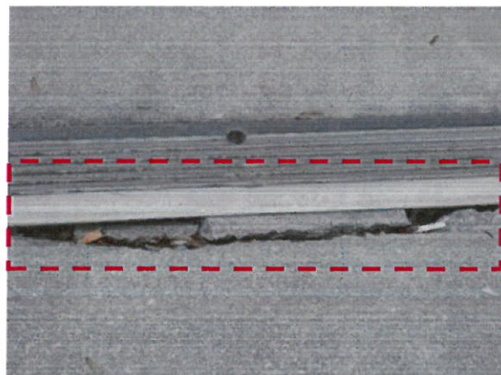
Photo 18: Full depth concrete spall along expansion joint on roof level of Parking Structure C
