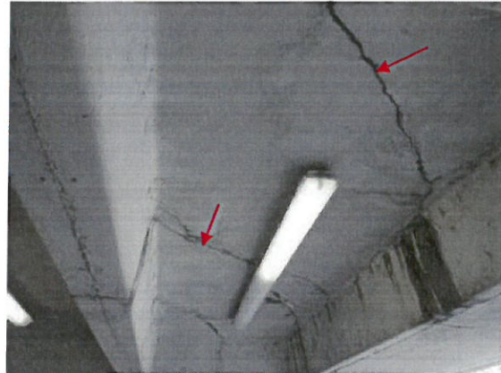
Photo 2: Underside view of cracks in the roof level slab
