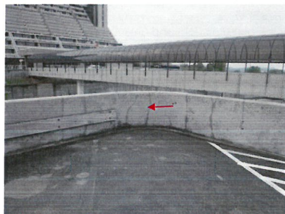
Photo 6: Cracks in perimeter walls
