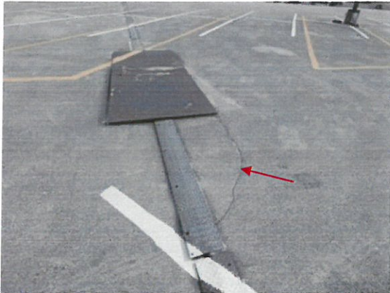
Photo 19: Concrete cracks parallel to expansion joint at roof level
