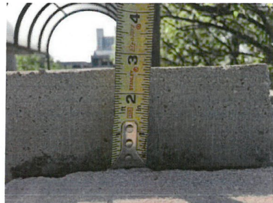
Photo 28: Vertical differential movement between two sides of the expansion joint on pedestrian bridge
