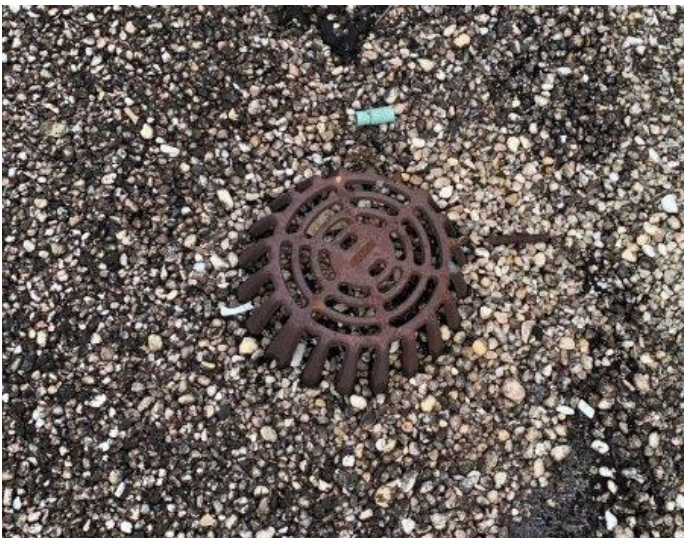
Roof Drain - Completely blocked
