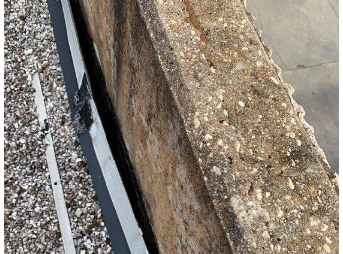
Roof Perimeter - Termination bar and coping flashing disconnected
