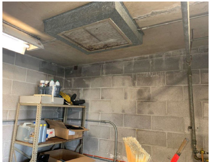
Interior (unpainted) walls - Efflorescence and water migration/staining
