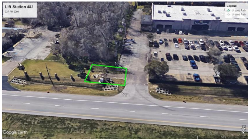
IV. 30. Lift Station #41 327 FM 2004 A
