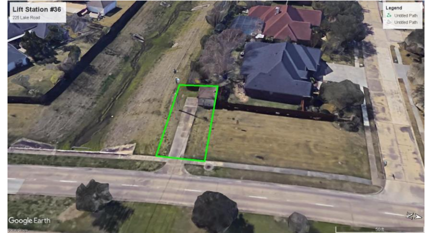
IV. 27. Lift Station #36 225 Lake Road
