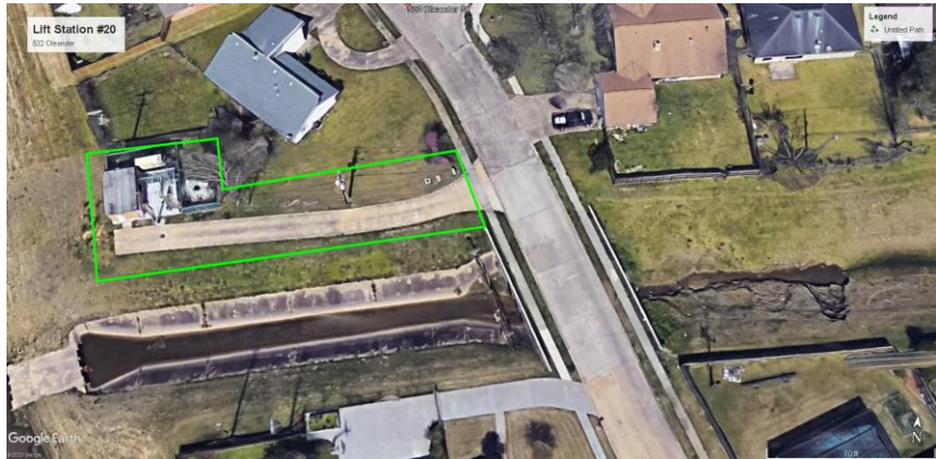
IV.14. Lift Station #20 532 Oleander
