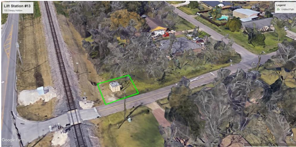
IV.9. Lift Station #13 100 Sleepy Hollow
