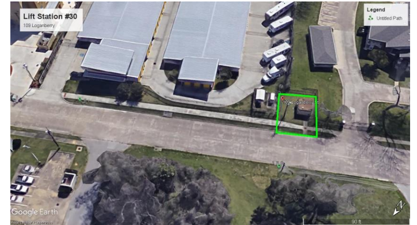
IV.23. Lift Station #30 109 Loganberry
