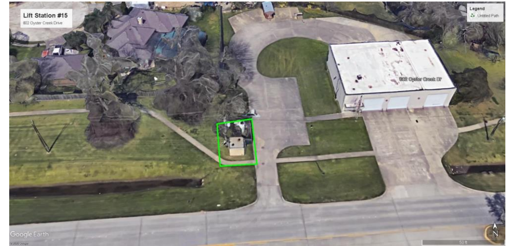
IV.11. Lift Station #15 602 Oyster Creek
