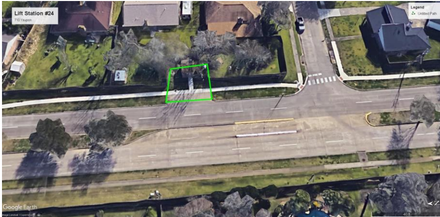
IV.17. Lift Station #24 710 Yaupon
