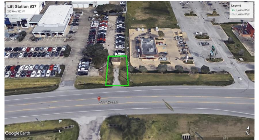
IV.28. Lift Station #37 212 HWY 332 W
