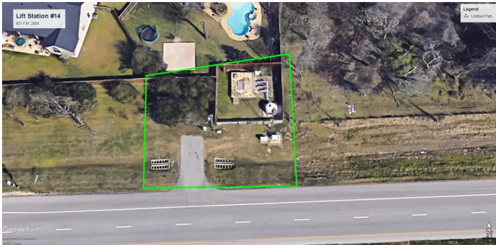
IV.10. Lift Station #14 501 HWY 2004
