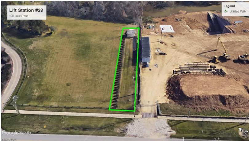
IV.21. Lift Station #28 198 Lake Road
