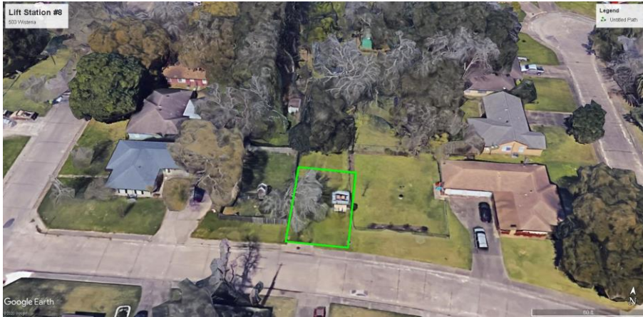
IV.5. Lift Station #8 503 Wisteria
