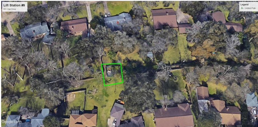
IV.6. Lift Station #9 531 Oak Drive
