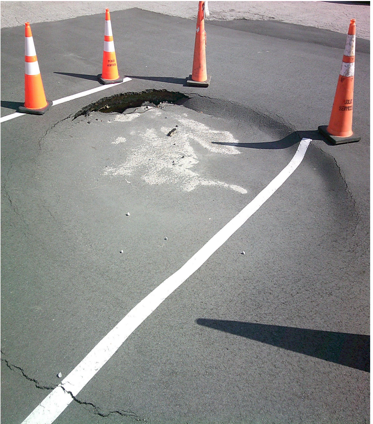
Figure 4: Image of the Sink Hole
