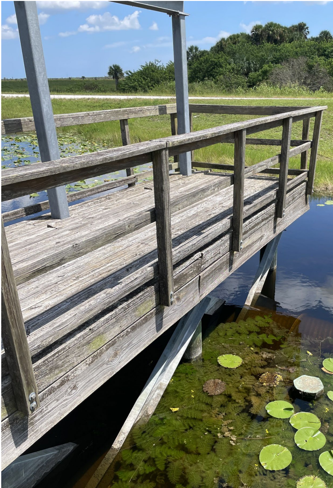
Figure 5: SJMCA – S-262 WALKWAY Platform at end of Walkway (east side)
