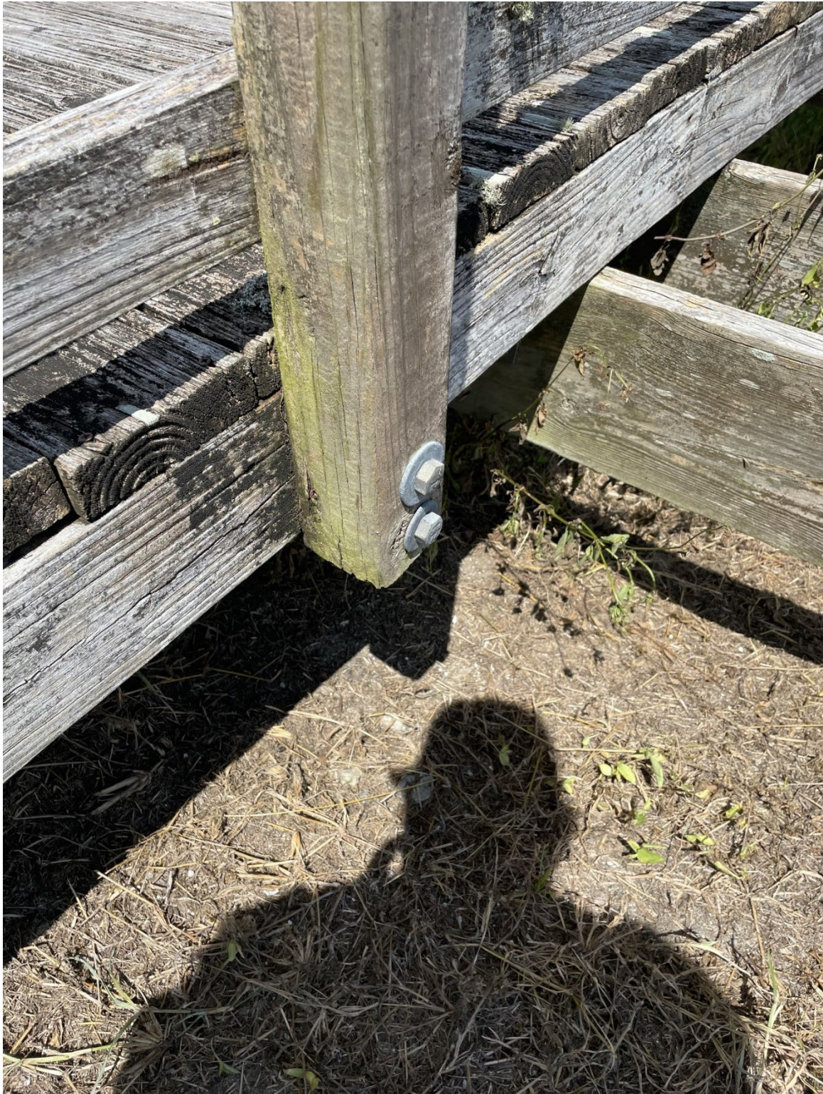
Figure 6: SJMCA – S-262 WALKWAY 4" by 4" Installation
