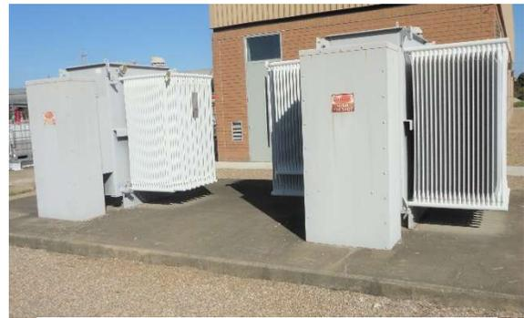
**Image 3: Compressor Building MV Transformers. Transformers were manufactured by Westinghouse in 1987.**
