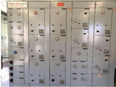
**Image 2: First Stage Equalization Building MCC-P1. GE 7700 Series Motor Control Center.**
