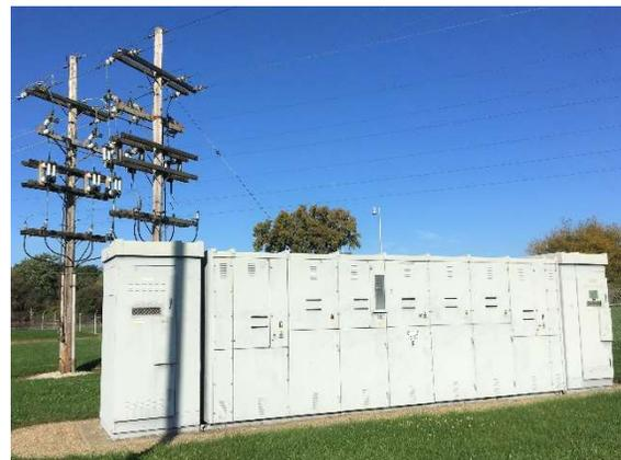
**Image 1: Plant incoming power with incoming pole mounted load break switches and 15kV Main Distribution Switchgear.**
