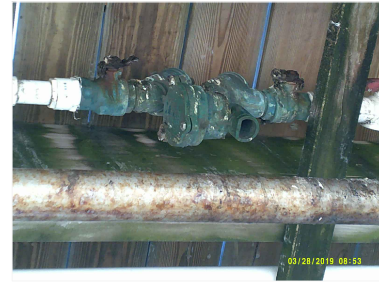
BENT 1: WATER BACK FLOW PREVENTER
