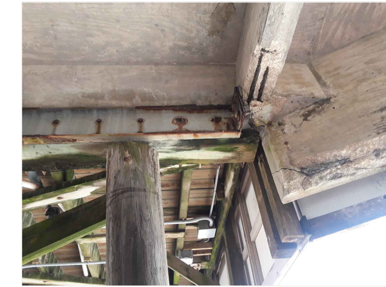
BENT 4: REPAIR CONCRETE BEAM CONNECTION
