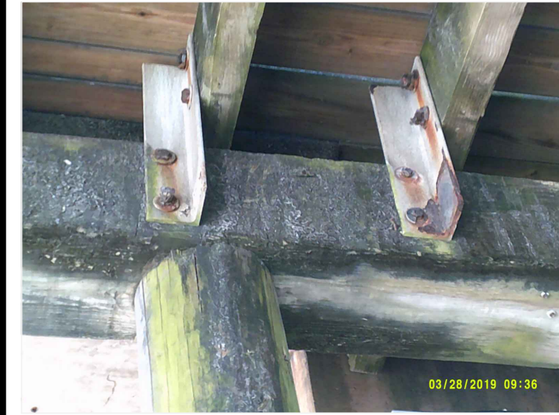
BENT 4: GALVANIZED BRACKETS
