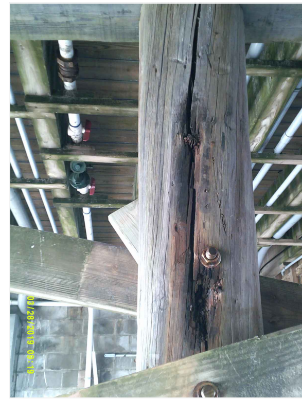
BENT 1: SPLIT 4th PILE in from North
