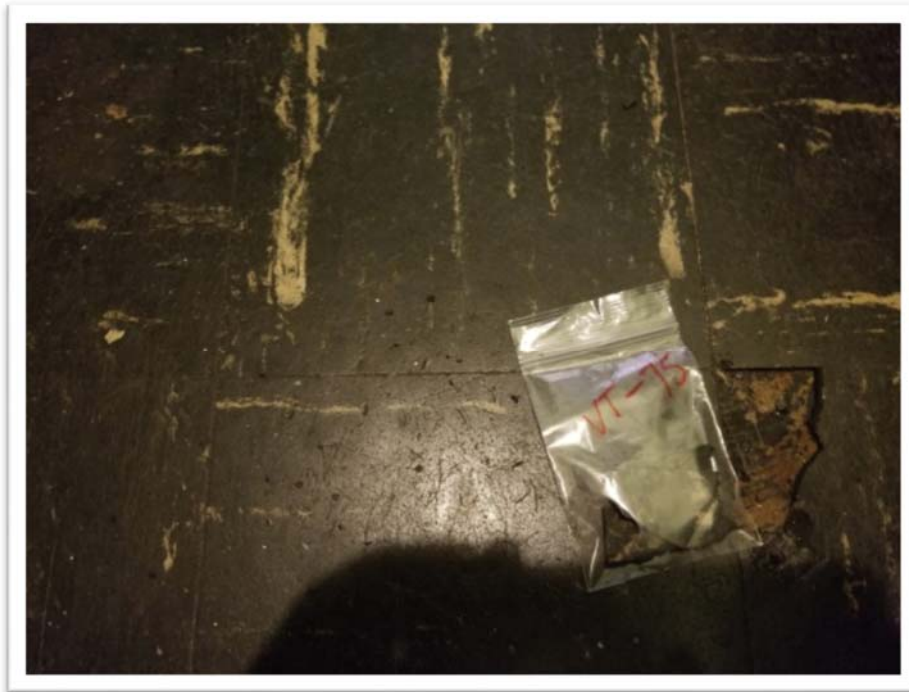
Photograph #12 Storage Closet by Medical Office, Sampling Point VT-75 – Additional View of Asbestos Containing 9”X9” Black with Cream Streaks VFT/Mastic.
