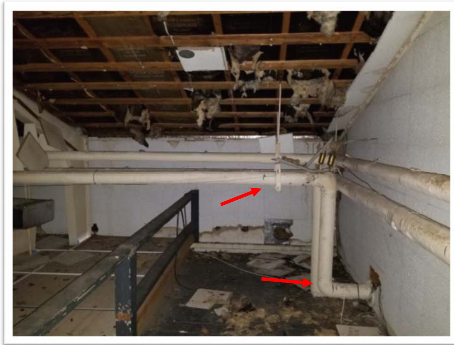
Photograph #23 Attic – View of TSI Pipe Wrap and Elbows. Elbows are 25% Chrysotile. Pipe Wrap is 25% to 30% Chrysotile and 15% to 18% Amosite.
