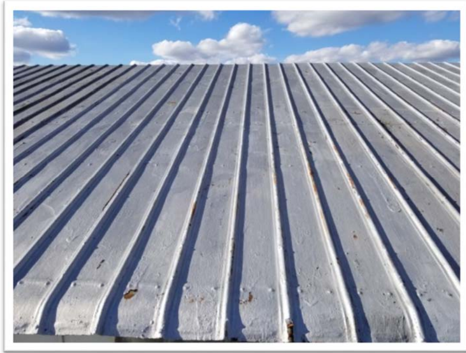
Photograph #21 Metal Roof – Surface Coating is 3% and 4% Chrysotile.
