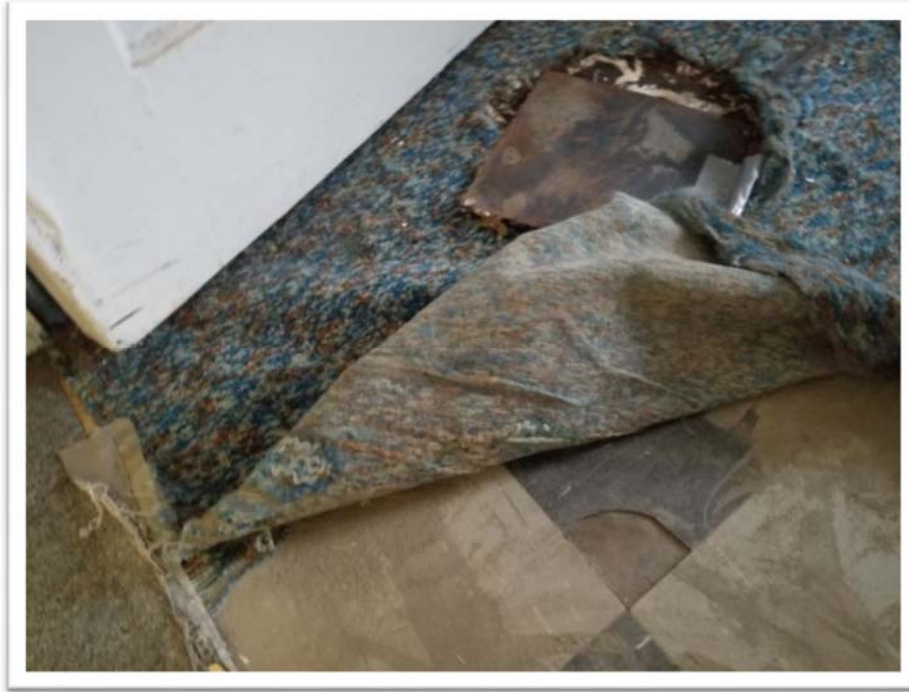
Photograph #11 Medical Office – 9”X9” Black with Cream Streaks and Gray VFT/Mastic (3%, 2% Chrysotile / 6% Chrysotile). See Appendix B, Figure 8 for Locations.
