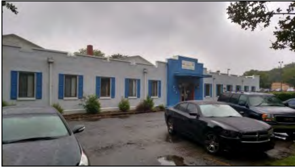
View of the northern side of the building.
