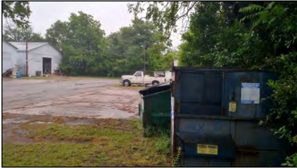
View of the southern property boundary from the northwest corner of the property.
