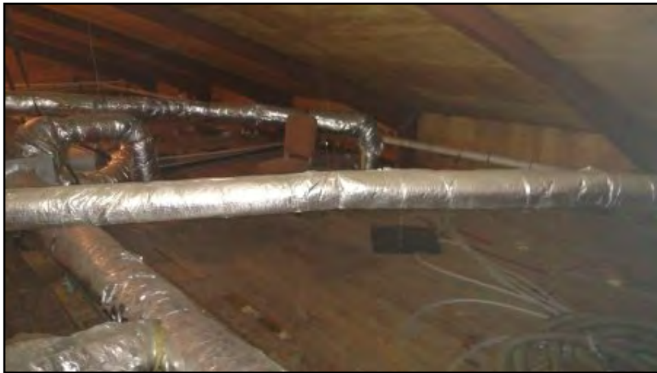
View of the attic.
