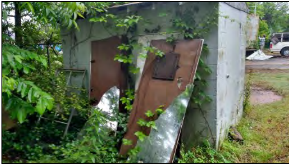
View of a shed near the southwest corner of the property.
