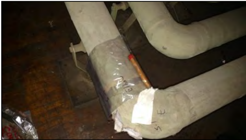
View of asbestos sample S-1 on the second floor of the building.
