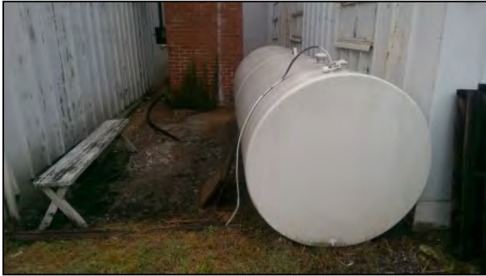
View of the AST on the southern side of the building.
