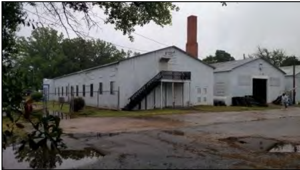
View of the northwest corner of the building.
