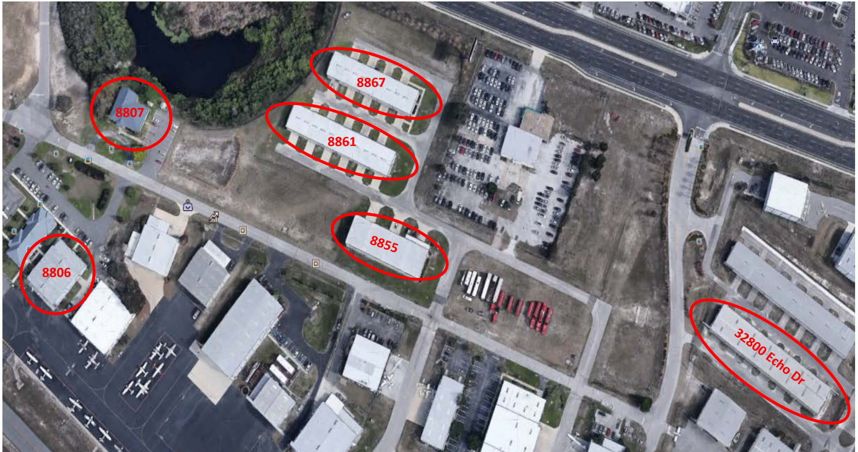
Aerial Photo of areas to be painted.
