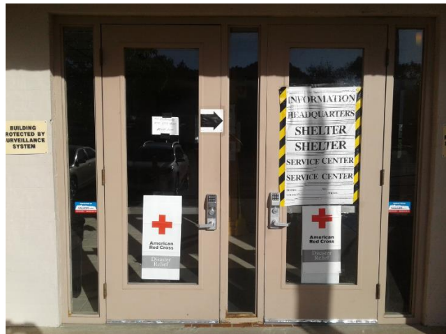
Doors 7 & 8 southwest entry
