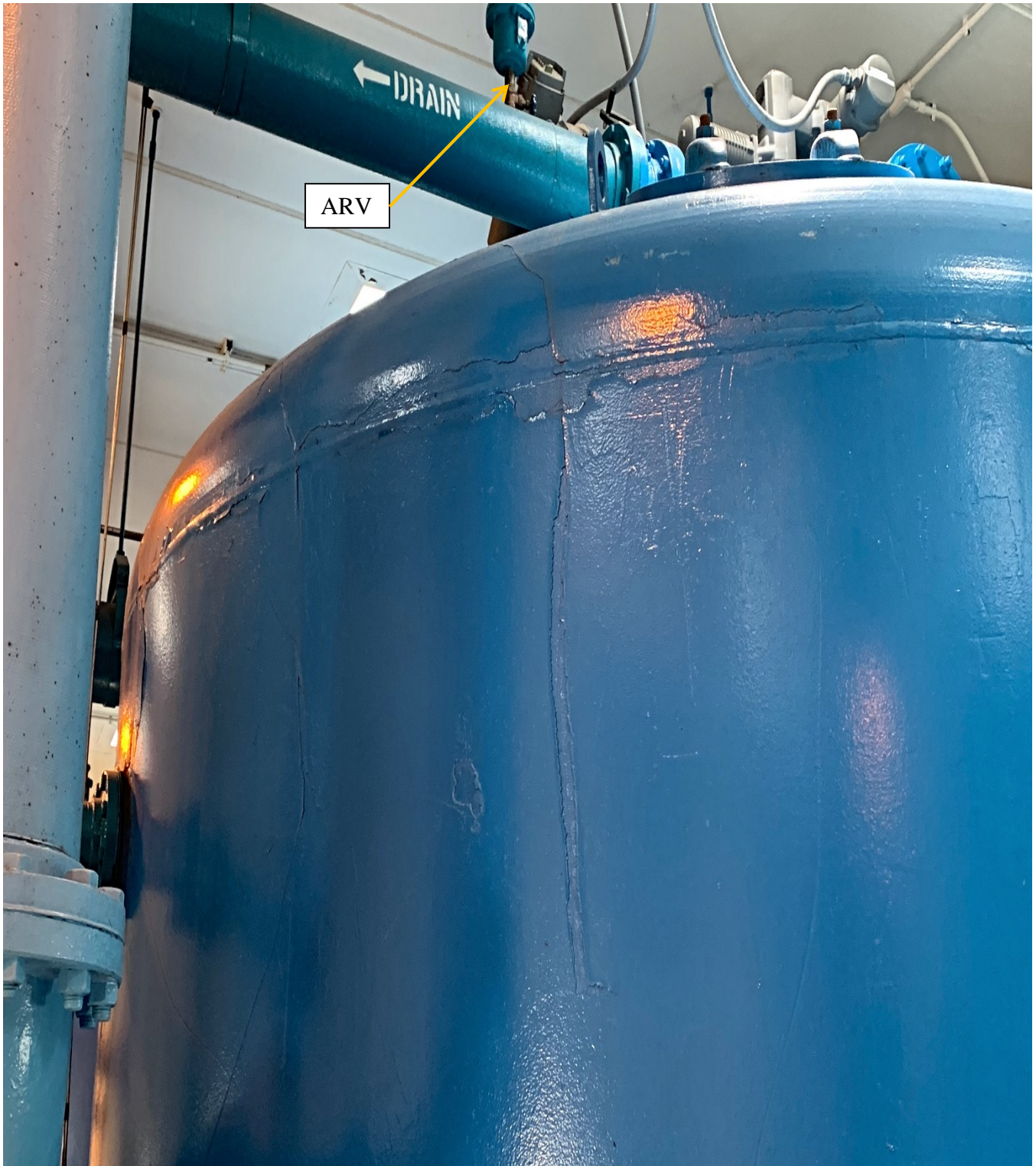
Figure 11 Air Release Valve (Side B only)
