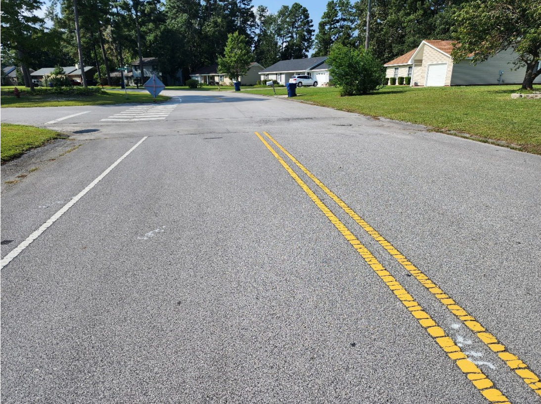
Figure 3: Existing Conditions Photos
