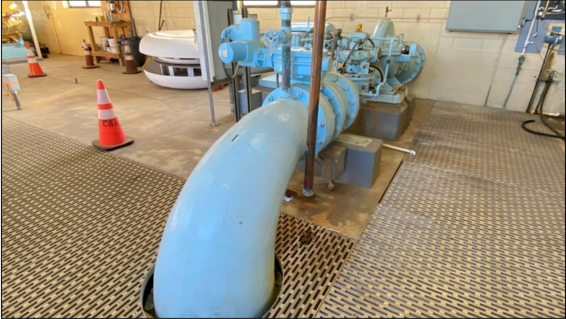
3 - View of blue paint on pipes
