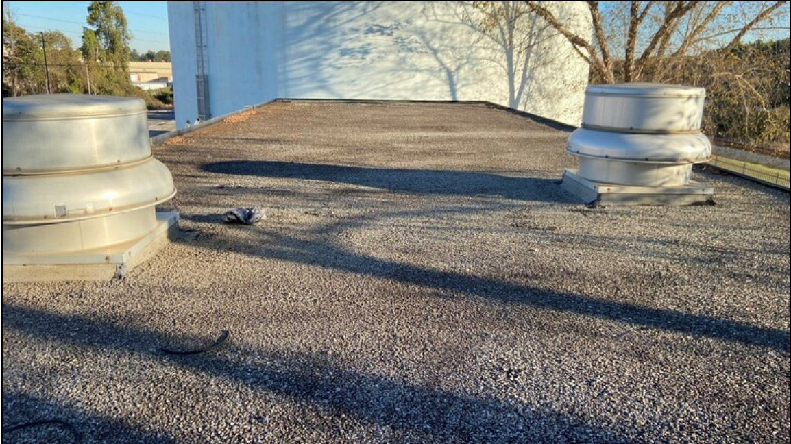
7 - View of the roof
