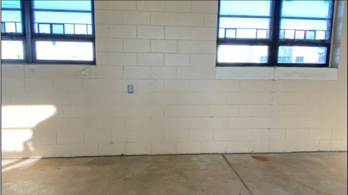
9 - View of yellow paint on CMU wall
