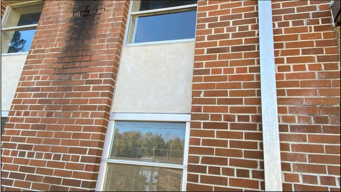
5 - View of the wall panels
