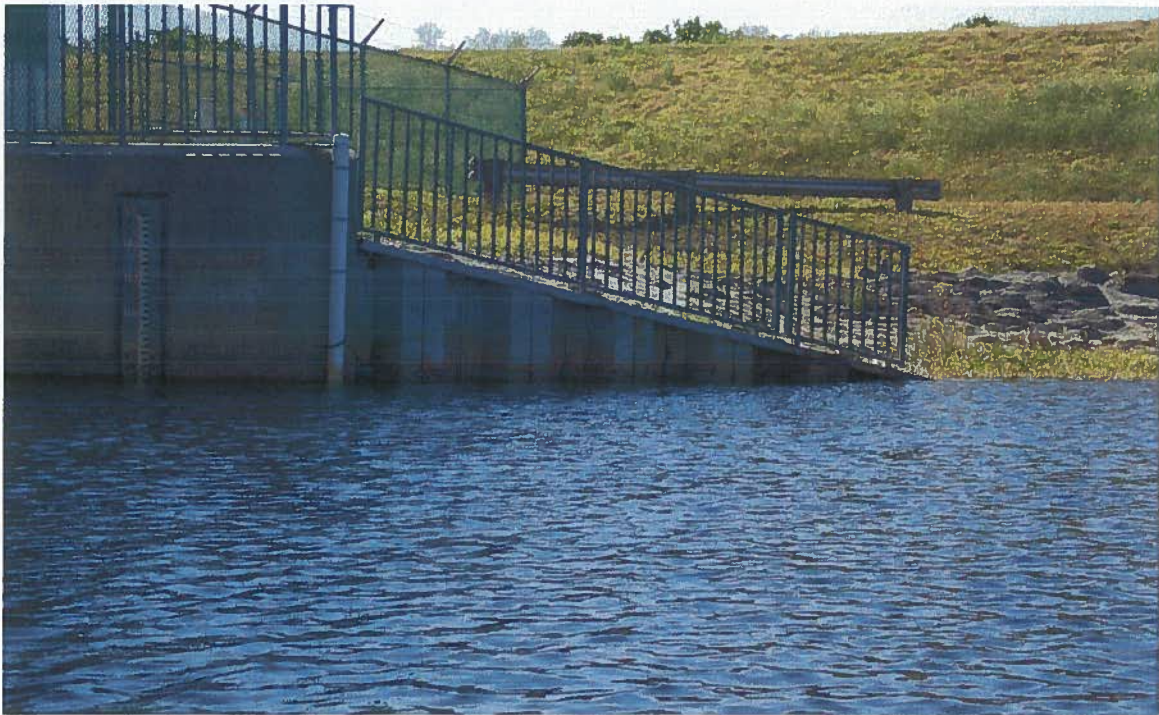
Upstream - South Steel Sheet Pile Wing Wall.
