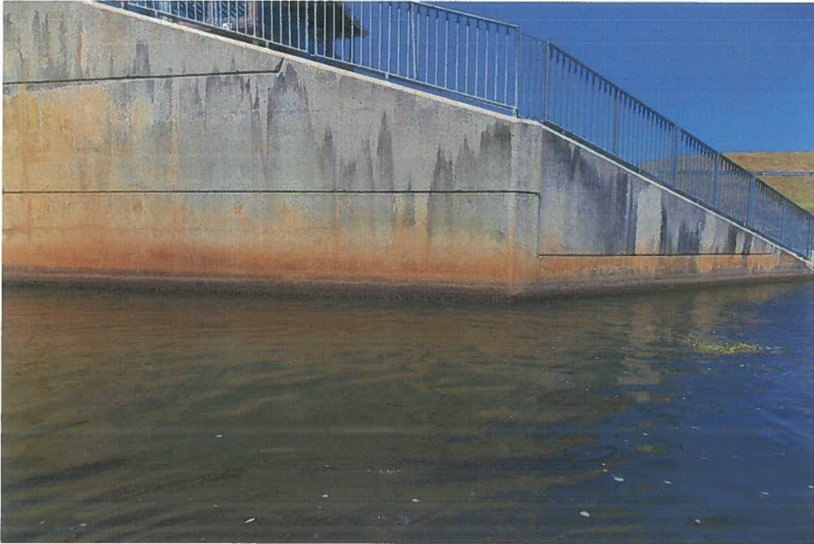
Downstream - North Mid-Panel and Wing Wall.
