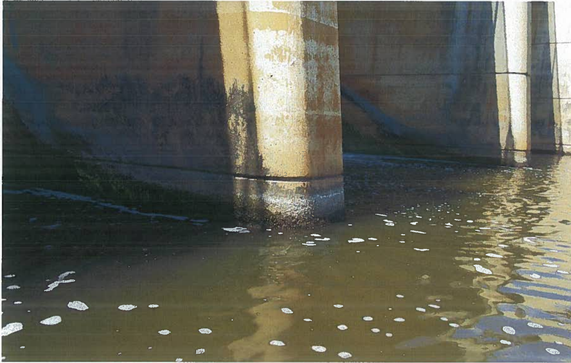
Downstream - South Bay - North Interior Wall and Mid-Bay North Interior Wall.
