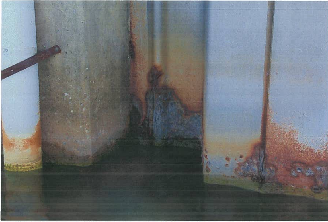
Upstream - South Wing Wall.
