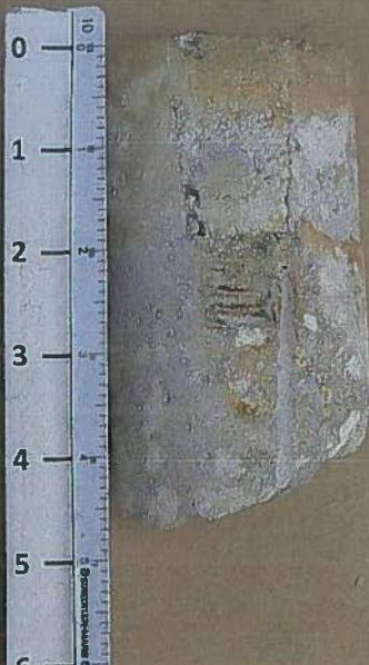
S-157 C-54 CANAL WATER CONTROL STRUCTURE Core No. 7
