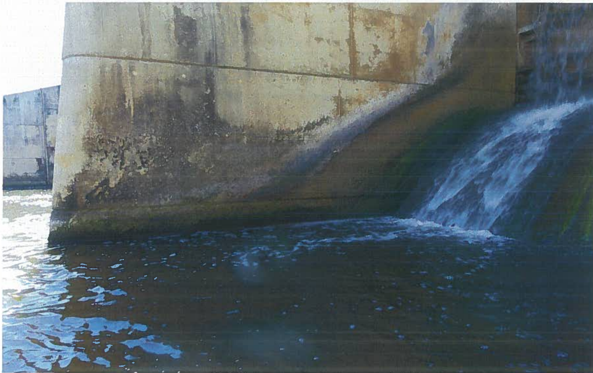
Downstream - North Bay, South Interior Wall.
