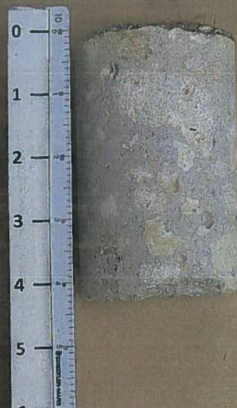
S-157 C-54 CANAL WATER CONTROL STRUCTURE Core No. 4
