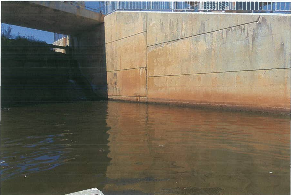
Downstream - North Bay Wall and Mid-Panel Wall.
