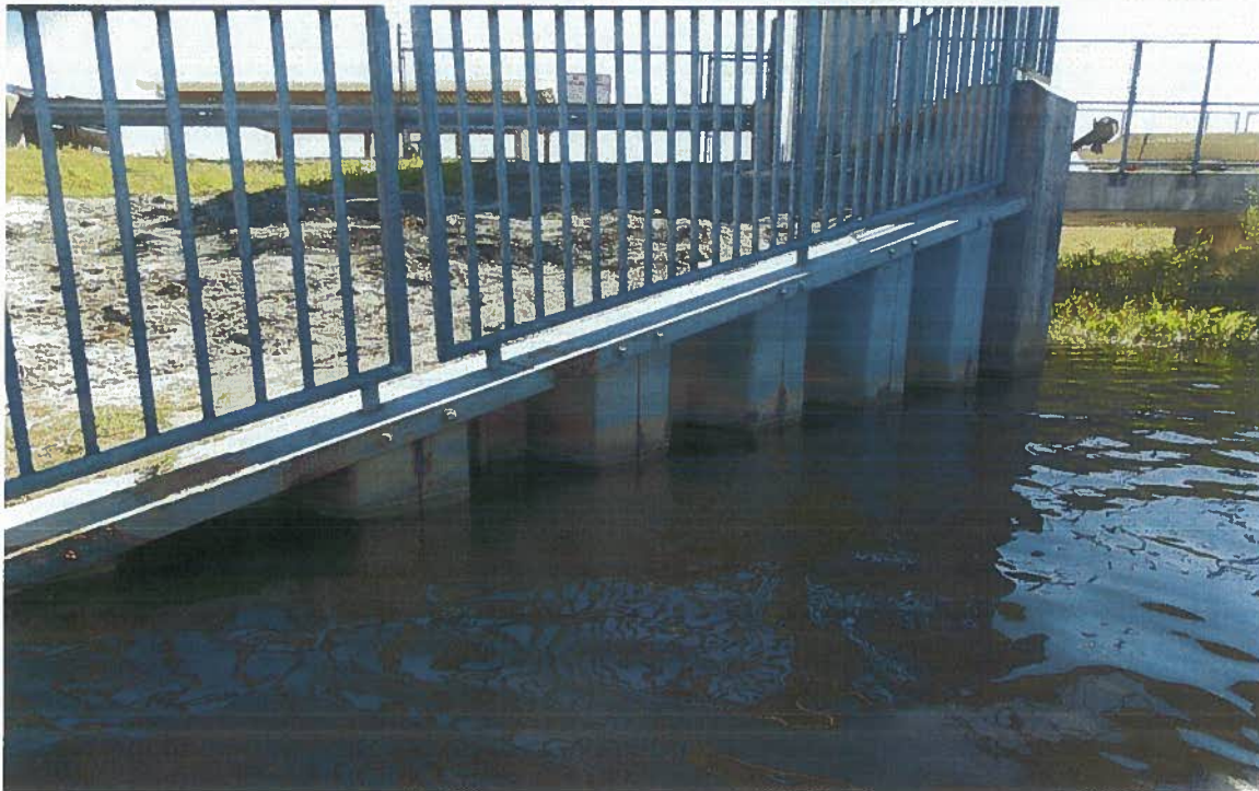
Upstream - North Steel Sheet Pile Wing Wall.
