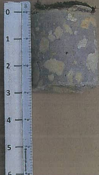
S-157 C-54 CANAL WATER CONTROL STRUCTURE INDIAN RIVER CTY, FL Core # 6
