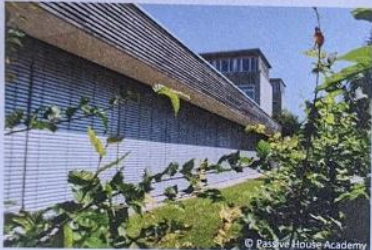
Blinds extended, preventing overheating
