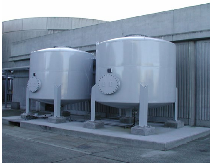
Figure 1. Adsorptive Media Installation Example
