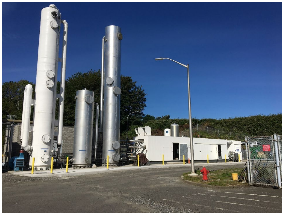
Figure 16. Typical Water Wash systems Installation
