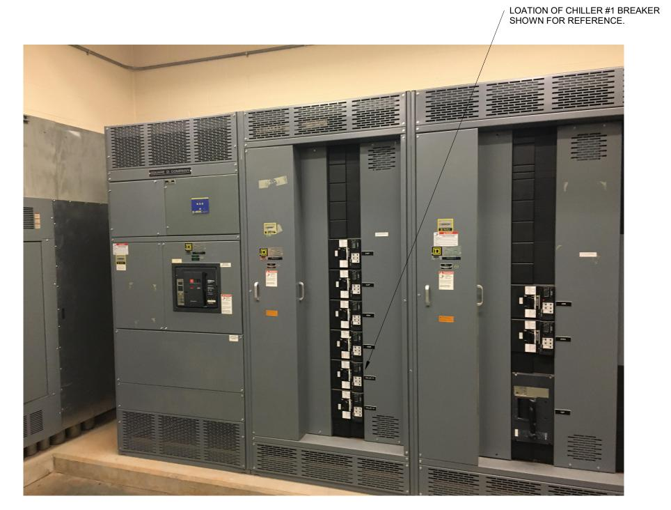
EXISTING SWITCHBOARD MSG FRONT ELEVATION
