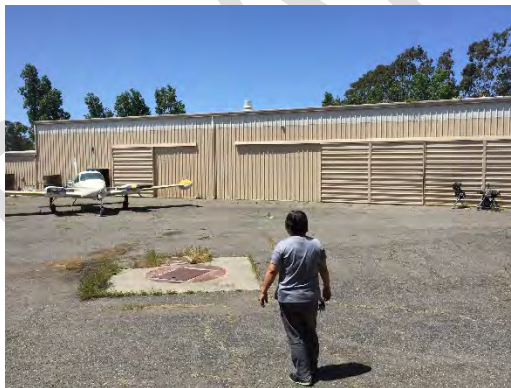
Hangar doors at Hangar A
