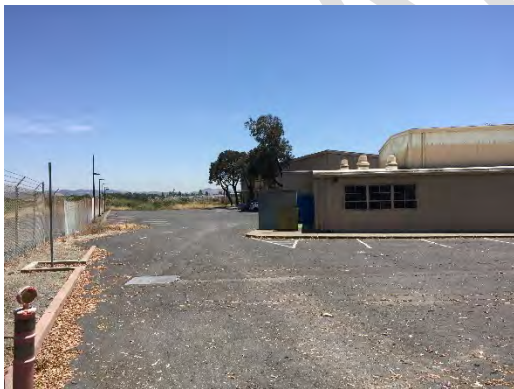
View of Hangar A at campus entry
