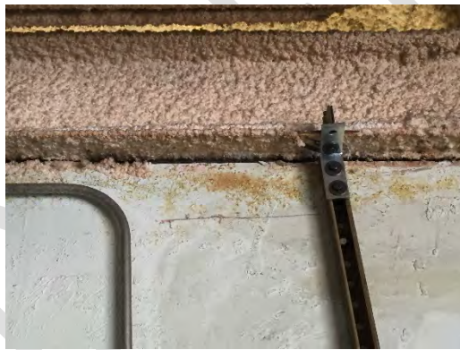
Structural reinforcement at informal partition between general classroom and Electrical Shop
