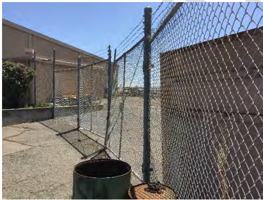
Fence between Ramp Area and Parking
