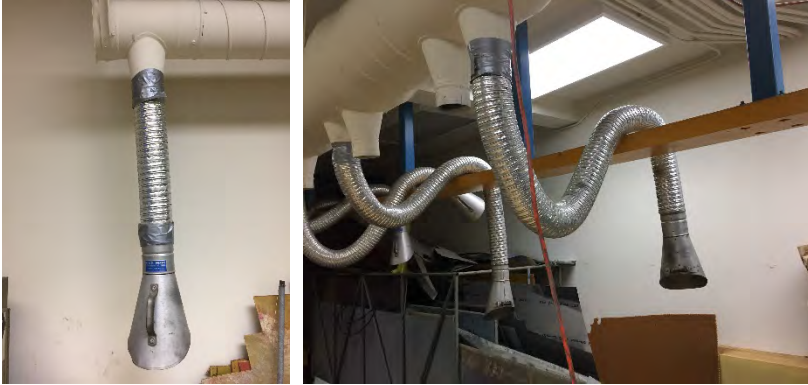
House-made suction heads (snorkel) in Composites Lab.
