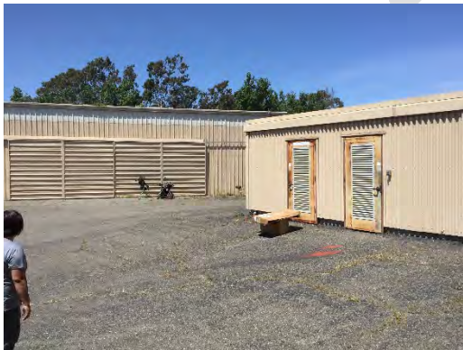
Hazmat storage shed in yard
