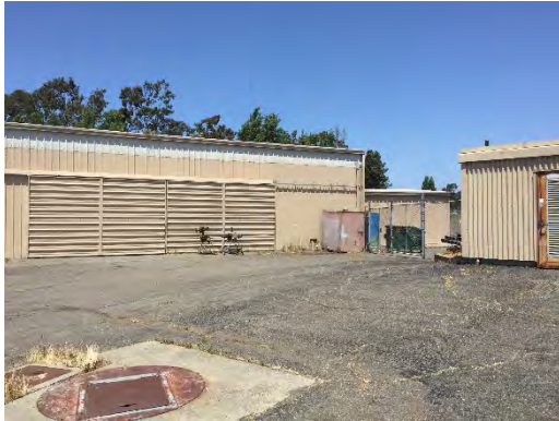
Paved yard, sump pump/lift station access cover
