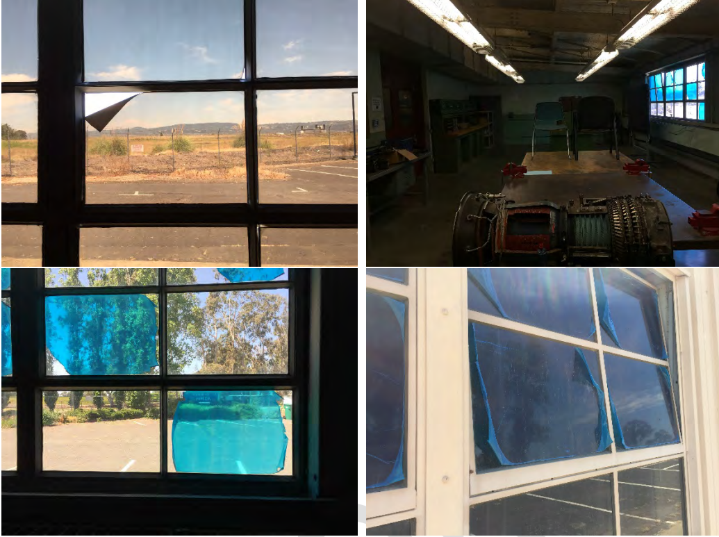
Glare control at Hangar A general classroom, views from interior and exterior
