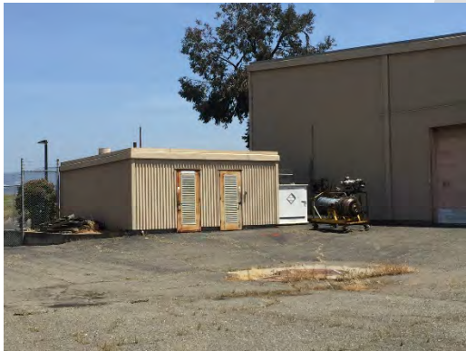
Chemical storage, jet fuel storage between Hangar A and Hangar B
