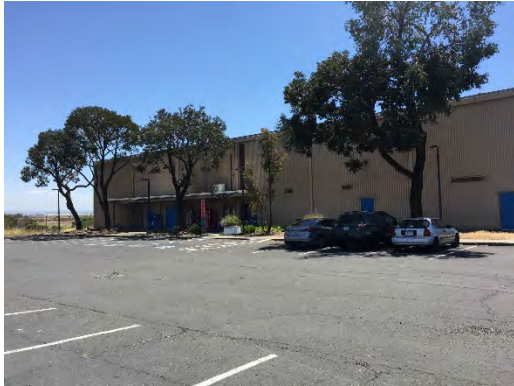
Front of Hangar B
