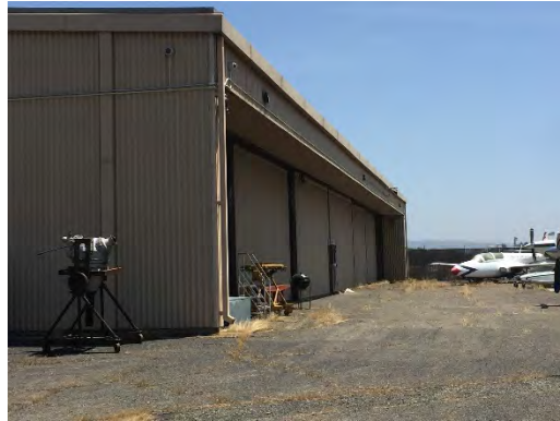
Two double hangar doors at Hangar B
