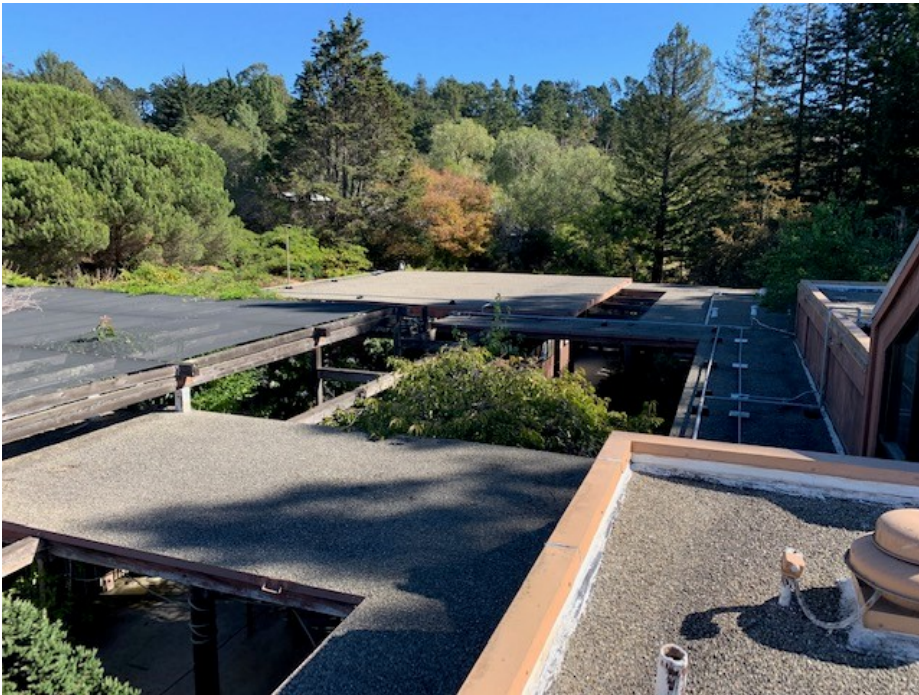
Photograph 16: View depicting the typical roof
