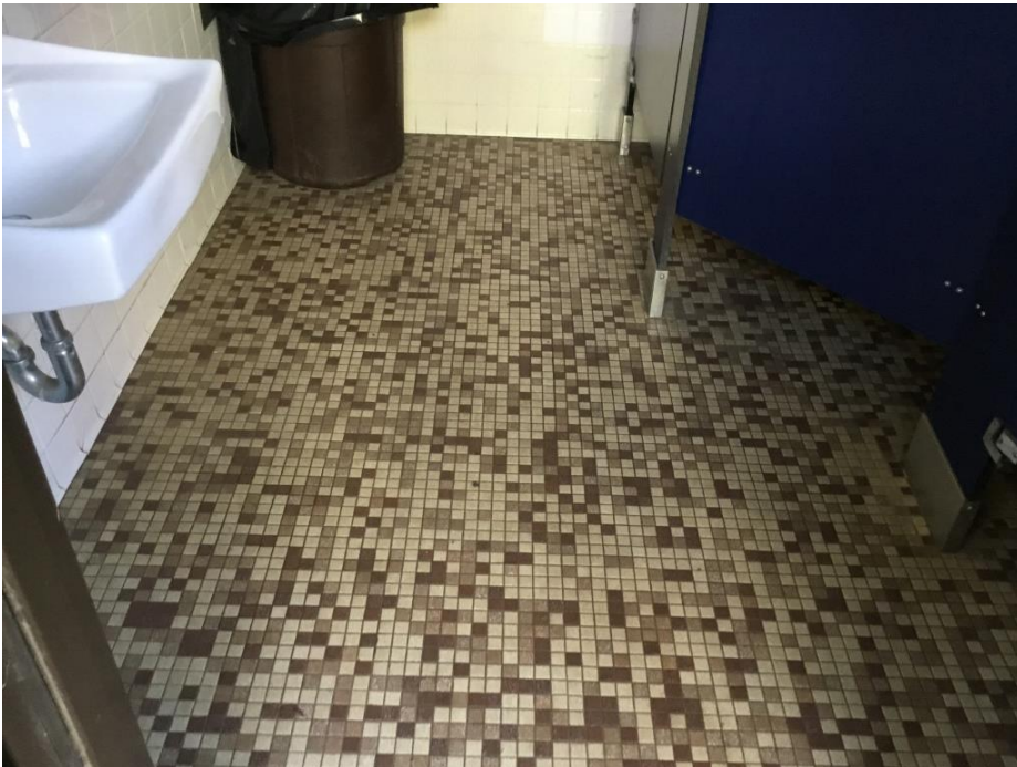
Photograph 14: View depicting the Restroom building interior.
