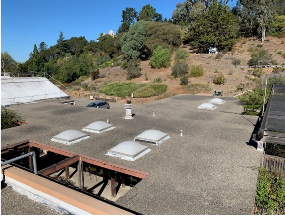
Photograph 15: View depicting the typical roof
