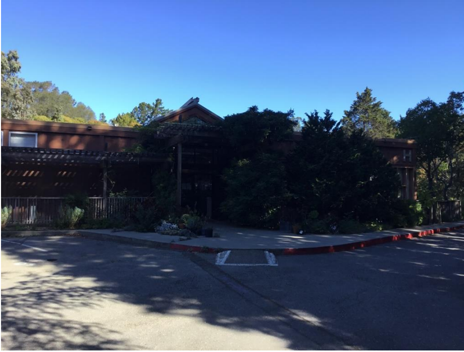
Photograph 1: View looking north at the Headhouse Building.
