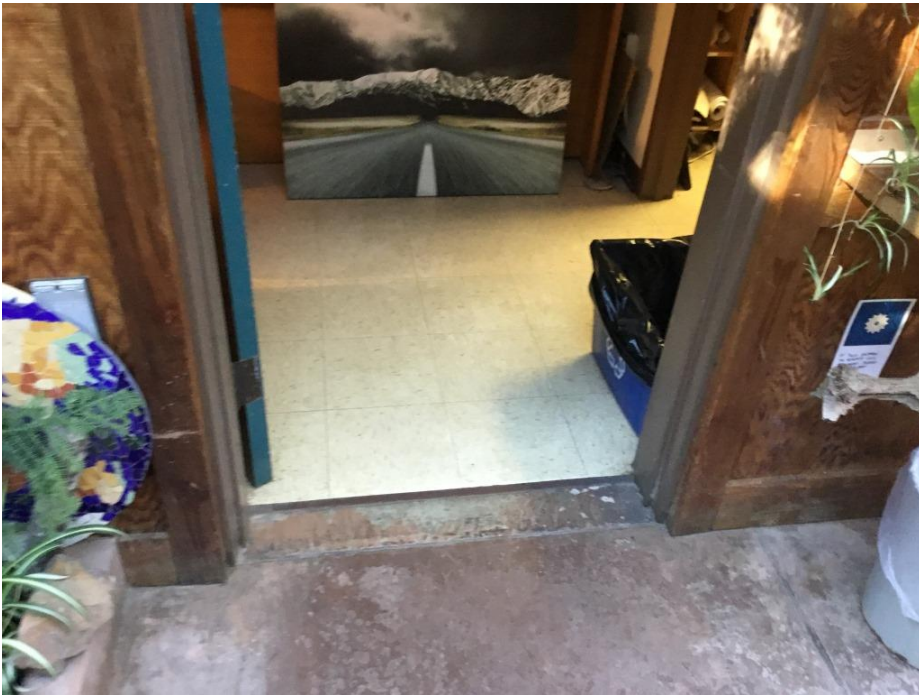
Photograph 2: View depicting entry to the Headhouse offices and janitor's closet.
