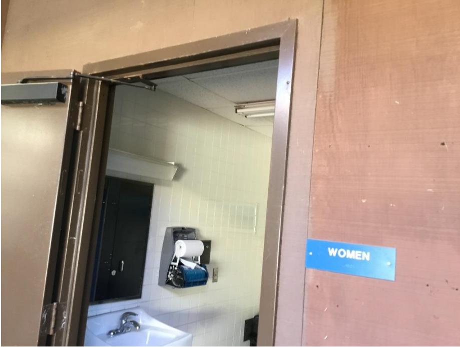
Photograph 13: View depicting the Restroom building interior.
