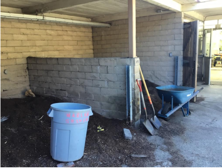
Photograph 9: View depicting the typical shed associated with the Boiler Room.
