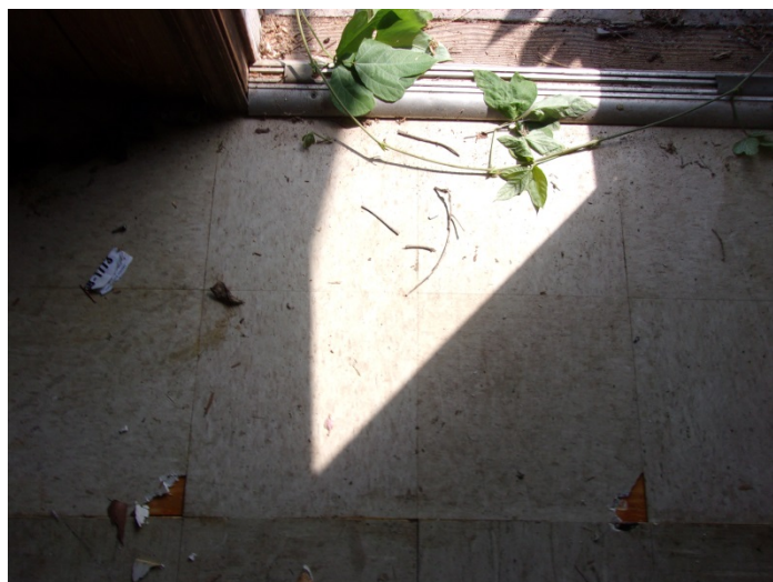
Photo 23 – 12" x 12" tan speckled floor tile & mastic in the apartment (patch)
