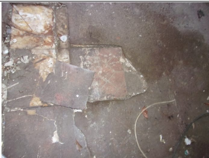
Photo 7 – Brown roll vinyl floor with no mastic over 12" x 12" floor tile & mastic in the grocery – top floor
