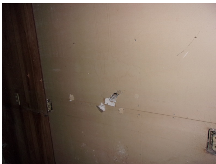
Photo 22 – Unfinished drywall throughout the doctor's office
