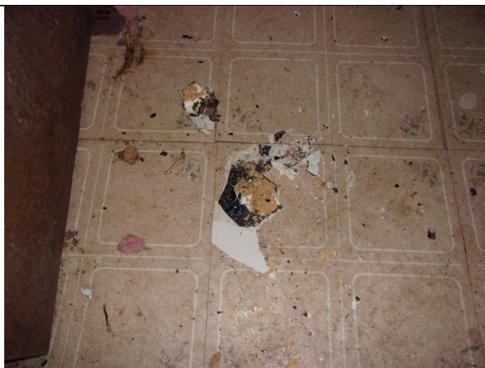
Photo 20 – 12" x 12" beige with flowers pattern self-stick floor tile over 2nd layer of floor tile & mastic in the doctor's office - 1/2 bathroom
