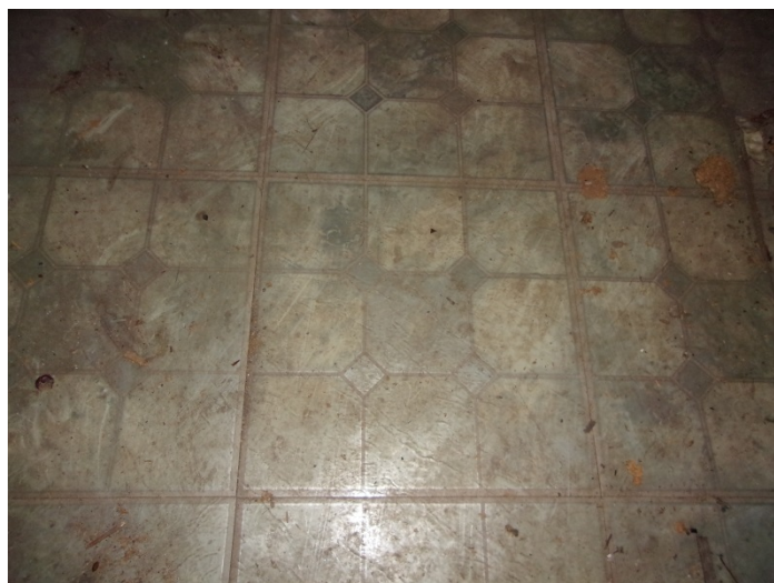
Photo 19 – 12"x 12" square pattern self-stick floor tile & mastic in the doctor's office - kitchen & full bathroom
