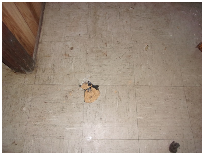
Photo 25 – 12" x 12" grey streaked floor tile & mastic in the apartment
