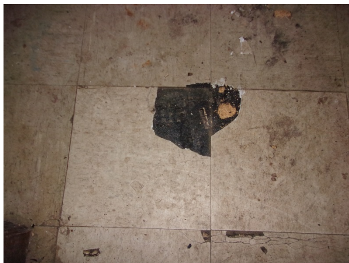
Photo 21 – 12" x 12" tan speckled floor tile & mastic in the doctor's office - front lobby & reception area
