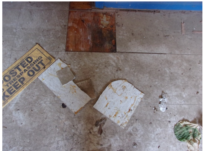
Photo 6 – 12" x 12" floor tile & mastic in the grocery top floor entrance
