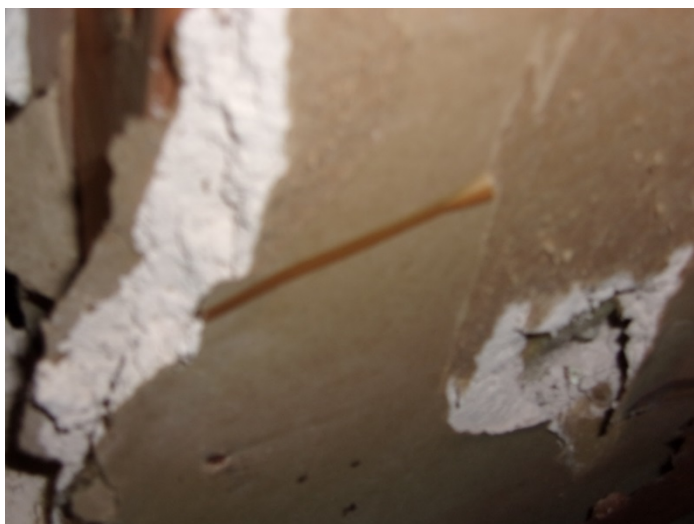
Photo 11 – Brown mastic behind wall panels in the grocery section bathroom & kitchen
