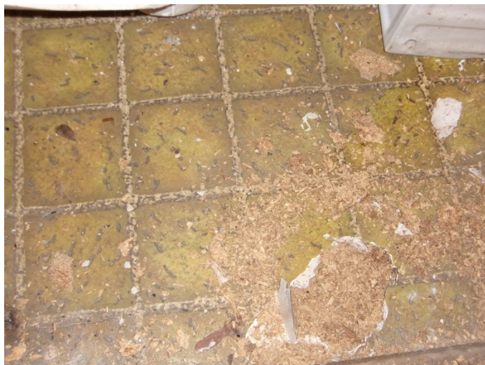
Photo 10 – Brown square roll pattern vinyl floor with no mastic in the grocery section bathrooms
