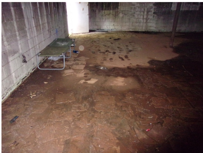
Photo 15 – 12" x 12" tan floor tile & black mastic in the basement
