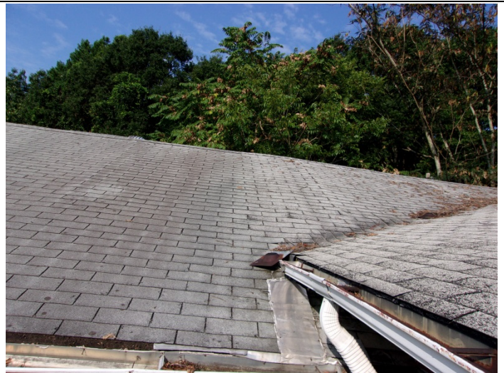
Photo 2 – Roof shingles & felt on the grocery, doctors office & apartment roofs
