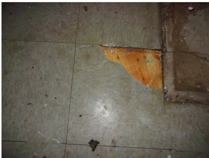
Photo 17 – 12" x 12" light green floor tile & mastic in the doctor's office - right side suite (top layer)
