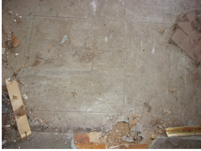
Photo 18 – 12" x 12" tan floor tile with fiberboard & black mastic in the doctor's office- right side suite (bottom layer & top layer throughout)
