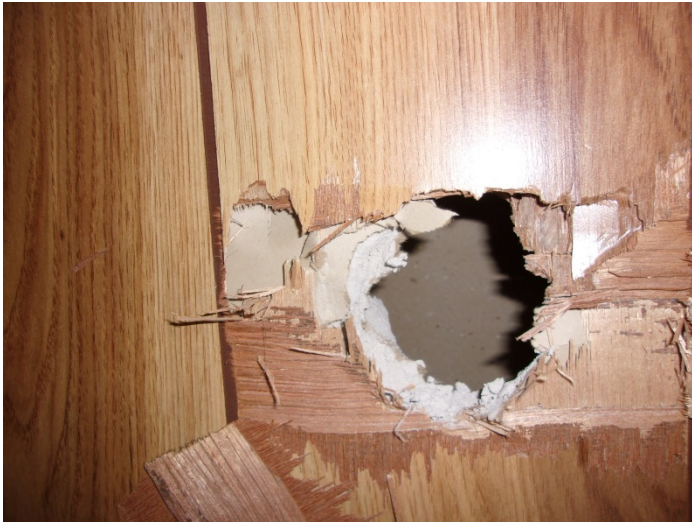
Photo 25 – Unfinished drywall under wooden wall panels in the apartment
