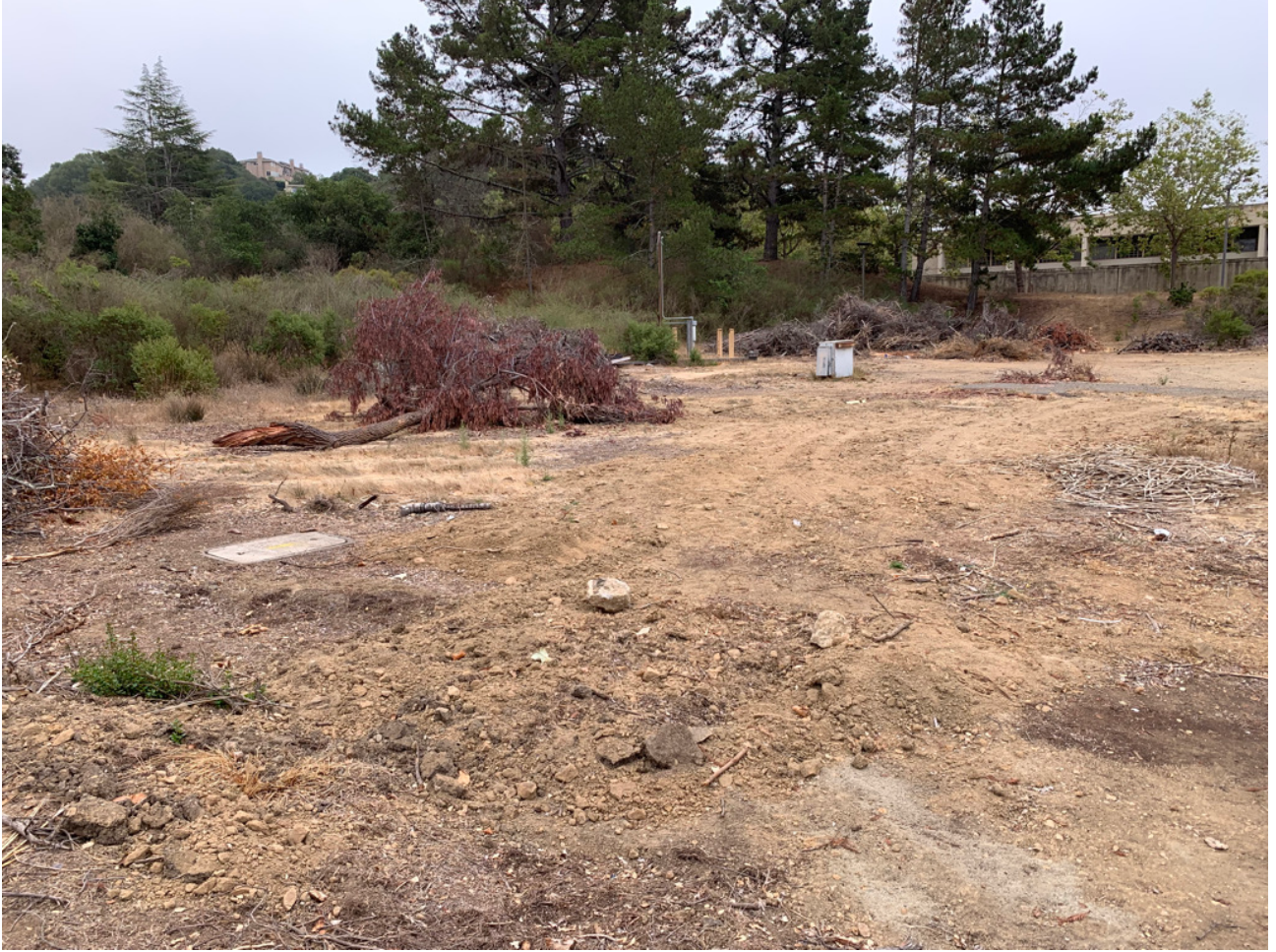
Figure 6: Photograph of the CDC site at the time of the geologic evaluation.
