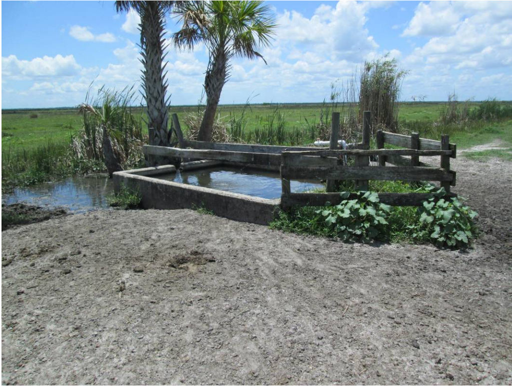
9. View of the concrete water trough and artesian well observed on the east central portion of the site.
