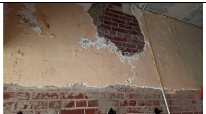
Picture 30 – *HA22 Plaster Wall Covering on Brick & Mortar Walls
