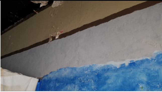
Picture 31 – *HA22 Plaster Wall Covering on Brick & Mortar Walls
