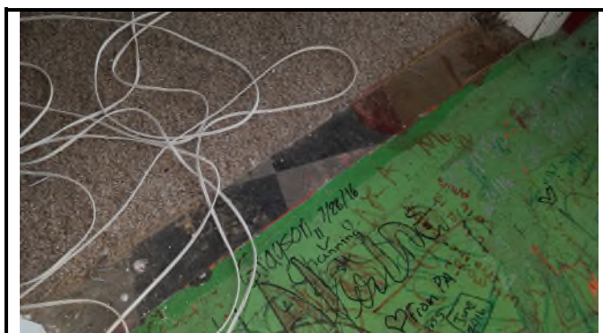
Picture 22 – *HA1 Painted 9x9 Floor Tiles w/Mastic and *HA1 Non-Painted 9x9 Floor Tiles 4% Chrysotile in Tile, 5% Chrysotile in Mastic
