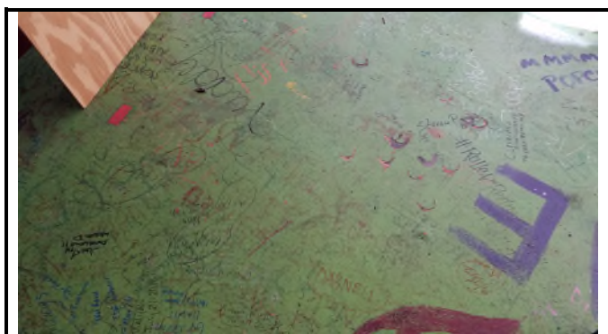
Picture 21 – *HA1 Painted 9x9 Floor Tiles w/Mastic 4% Chrysotile in Tile, 5% Chrysotile in Mastic
