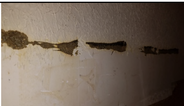
Picture 41 – *HA60 Wall Mastic 5% Chrysotile Present in Mastic
