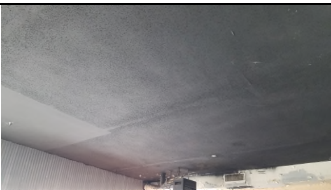
Picture 35 – *HA31 Sprayed Ceiling Texture
