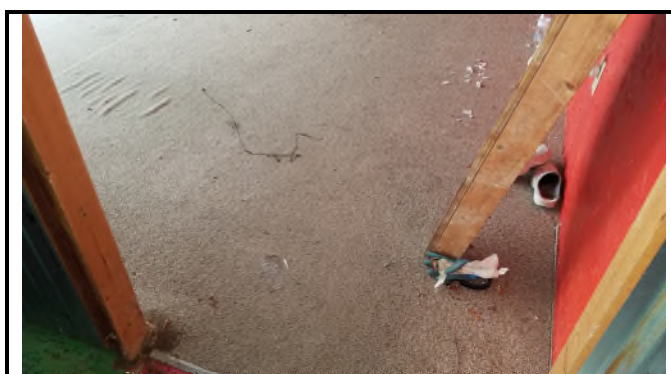
Picture 22 – *HA1 Painted 9x9 Floor Tiles w/Mastic and *HA1 Non-Painted 9x9 Floor Tiles 4% Chrysotile in Tile, 5% Chrysotile in Mastic
