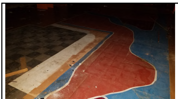
Picture 21 – *HA1 Painted 9x9 Floor Tiles w/Mastic 4% Chrysotile in Tile, 5% Chrysotile in Mastic
