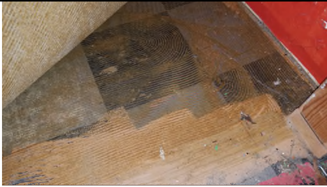
Picture 25 – *HA1 Non-Painted 9x9 Floor Tiles w/Mastic underneath *HA2 Carpet w/Mastic 4% Chrysotile in Tile, 5% Chrysotile in Mastic
