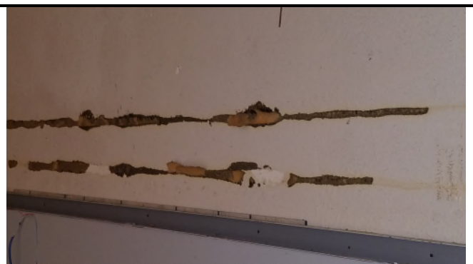
Picture 42 – *HA60 Wall Mastic 5% Chrysotile Present in Mastic
