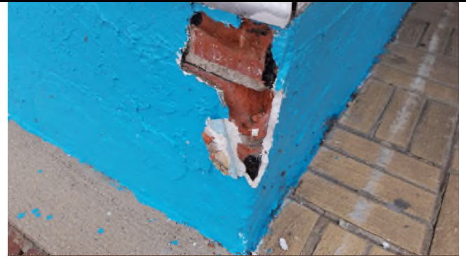
Picture 50 – *HA90 Exterior Wall Covering 7% Chrysotile Present in Black Adhesive-Like Material
