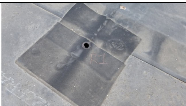
Picture 47 – *HA80 Roofing Materials – Core Sample R1
