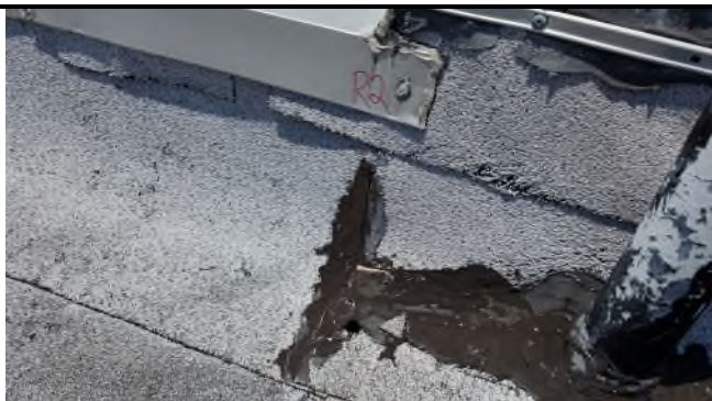
Picture 79 – *HA80 Roofing Materials – Core Sample R2
