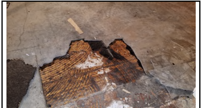
Picture 58 – *HA2 9x9 Floor Tiles w/Mastic 3% Chrysotile Present in Floor Tiles Mastic NAD
