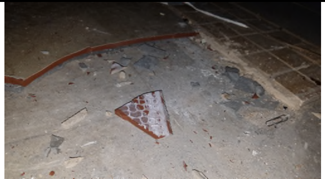
Picture 26 – *HA1 12x12 Floor Tiles w/Mastic (underneath Ceramic Tile)
