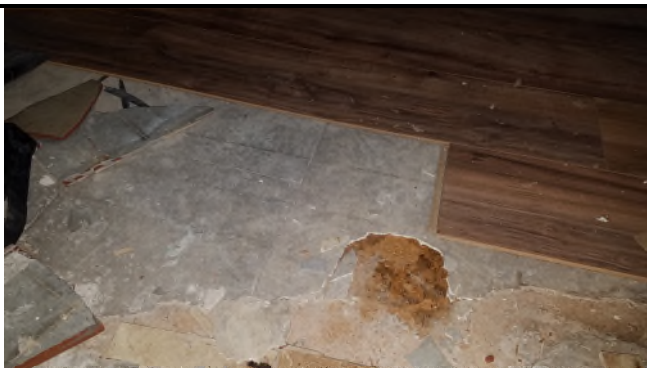
Picture 23 – *HA1 12x12 Floor Tiles w/Mastic (underneath Laminate Flooring)
