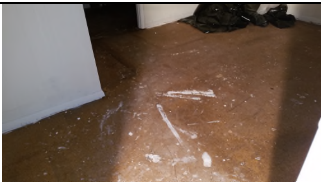
Picture 57 – *HA2 9x9 Floor Tiles w/Mastic 3% Chrysotile Present in Floor Tiles Mastic NAD
