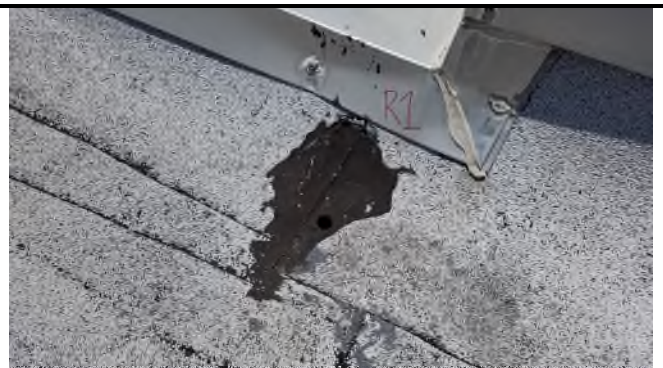
Picture 78 – *HA80 Roofing Materials – Core Sample R1
