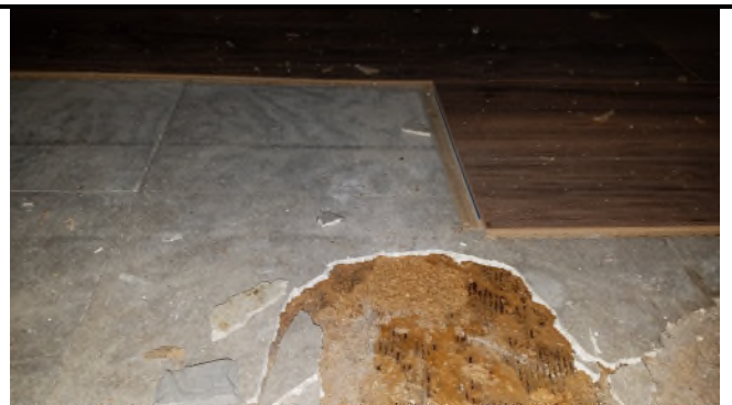
Picture 24 – *HA1 12x12 Floor Tiles w/Mastic (underneath Laminate Flooring)
