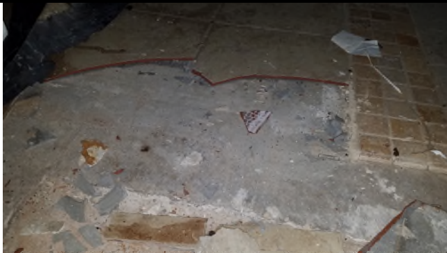
Picture 25 – *HA1 12x12 Floor Tiles w/Mastic (underneath Ceramic Tile)
