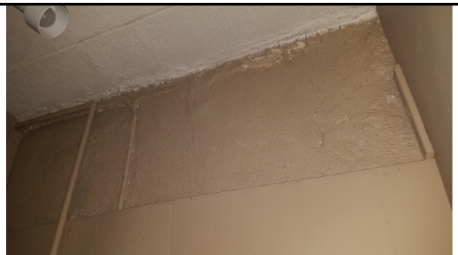
Picture 30 – *HA21 Interior Stucco Wall Covering 2% Chrysotile in Joint Compound-Like Material
