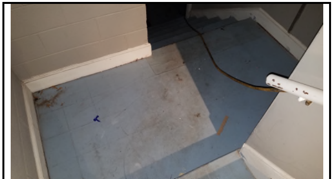
Picture 58 – *HA2 9x9 Floor Tiles w/Mastic 3% Chrysotile Present in Floor Tiles Mastic NAD
