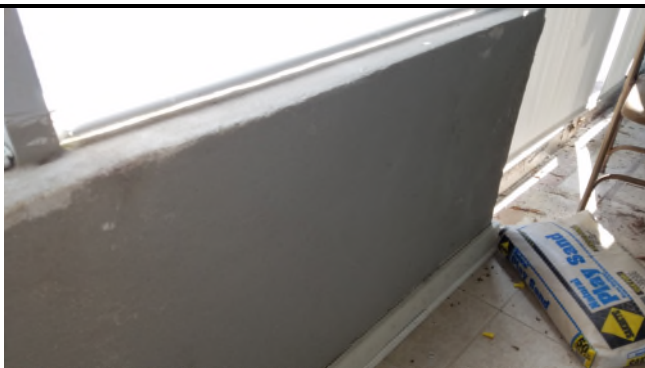
Picture 29 – *HA21 Interior Stucco Wall Covering 2% Chrysotile in Joint Compound-Like Material
