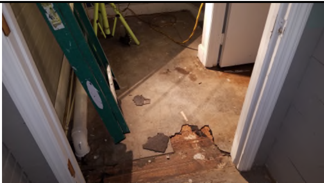
Picture 57 – *HA2 9x9 Floor Tiles w/Mastic 3% Chrysotile Present in Floor Tiles Mastic NAD
