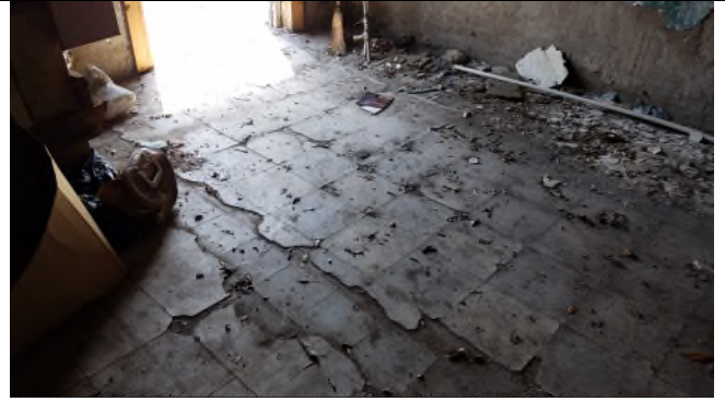
Picture 8 – *HA1 9x9 Floor Tiles, *HA2 9x9 Floor Tiles and *HA3 12x12 Floor Tiles w/Mastic (3 Layers)
