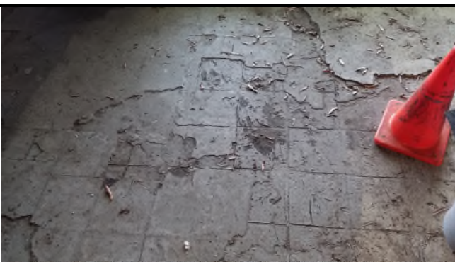
Picture 15 – *HA1 9x9 Floor Tiles, *HA2 9x9 Floor Tiles and *HA3 12x12 Floor Tiles w/Mastic (3 Layers)
