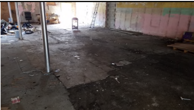
Picture 9 – *HA1 9x9 Floor Tiles, *HA2 9x9 Floor Tiles and *HA3 12x12 Floor Tiles w/Mastic (3 Layers)
