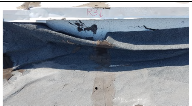
Picture 34 – Roofing Materials – Core Sample R3
