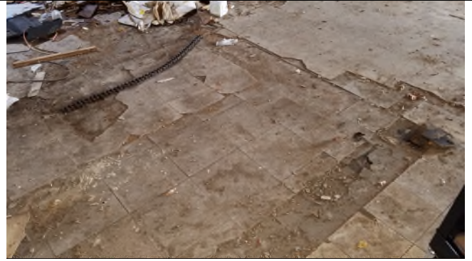
Picture 14 – *HA1 9x9 Floor Tiles, *HA2 9x9 Floor Tiles and *HA3 12x12 Floor Tiles w/Mastic (3 Layers)
