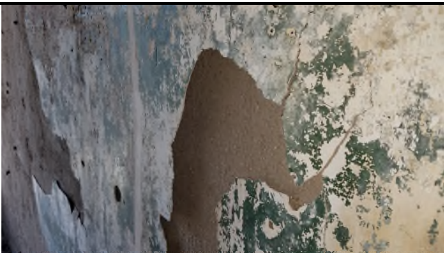
Picture 19 – *HA1 9x9 Floor Tiles, *HA2 9x9 Floor Tiles and *HA3 12x12 Floor Tiles w/Mastic (3 Layers)
