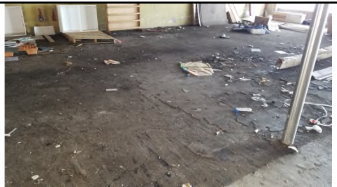
Picture 14 – *HA1 9x9 Floor Tiles, *HA2 9x9 Floor Tiles and *HA3 12x12 Floor Tiles w/Mastic (3 Layers)
