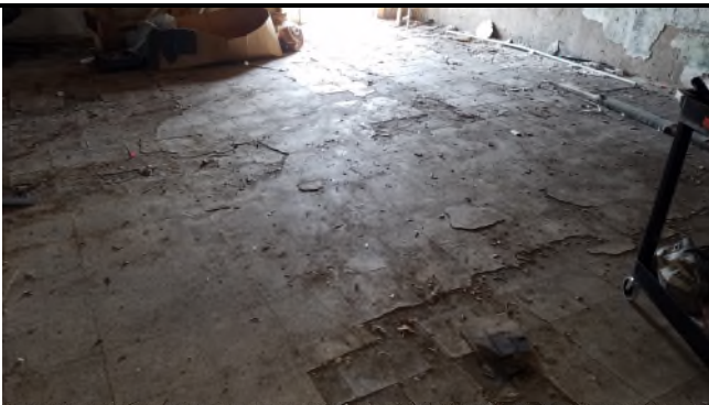
Picture 9 – *HA1 9x9 Floor Tiles, *HA2 9x9 Floor Tiles and *HA3 12x12 Floor Tiles w/Mastic (3 Layers)
