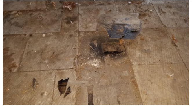
Picture 20 – *HA1 9x9 Floor Tiles, *HA2 9x9 Floor Tiles and *HA3 12x12 Floor Tiles w/Mastic (3 Layers)
