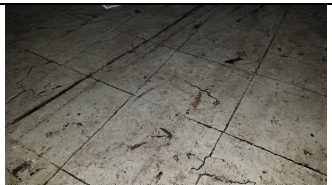
Picture 16 – *HA1 9x9 Floor Tiles, *HA2 9x9 Floor Tiles and *HA3 12x12 Floor Tiles w/Mastic (3 Layers)
