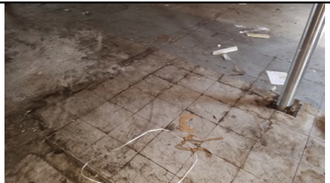
Picture 8 – *HA1 9x9 Floor Tiles, *HA2 9x9 Floor Tiles and *HA3 12x12 Floor Tiles w/Mastic (3 Layers)
