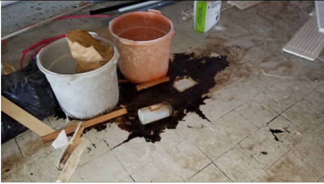
Picture 19 – *HA1 9x9 Floor Tiles, *HA2 9x9 Floor Tiles and *HA3 12x12 Floor Tiles w/Mastic (3 Layers)
