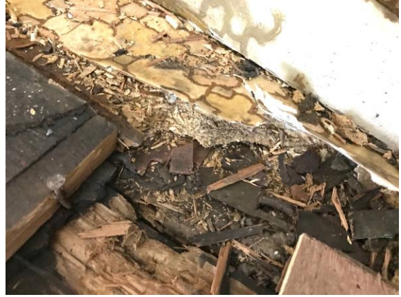
1209 Island Home Bathroom – 4 layers patterned vinyl sheet flooring & reddish brown VFT underneath
