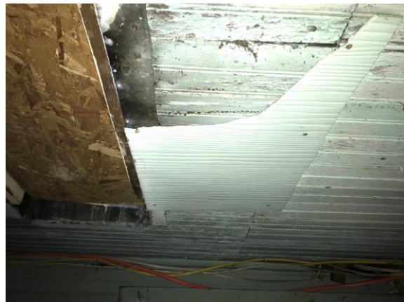
1209 Island Home Basement – wall-mounted & ceiling-mounted Transite panels
