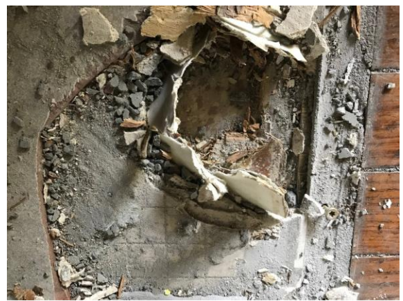
ACM VFT & vinyl under ceramic tile in Kitchen
