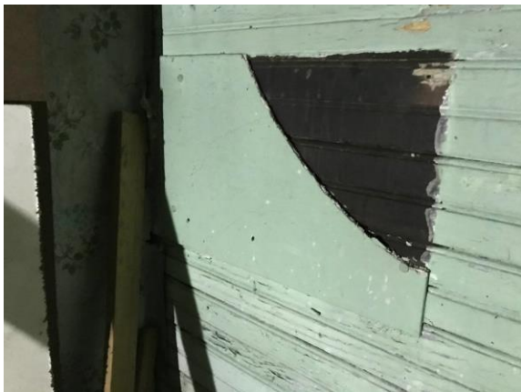
1209 Island Home Basement – wall-mounted & ceiling-mounted Transite panels
