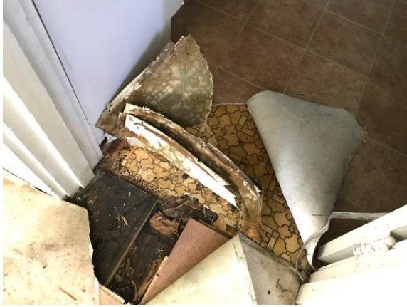
1209 Island Home Bathroom – 4 layers patterned vinyl sheet flooring & reddish brown VFT underneath
