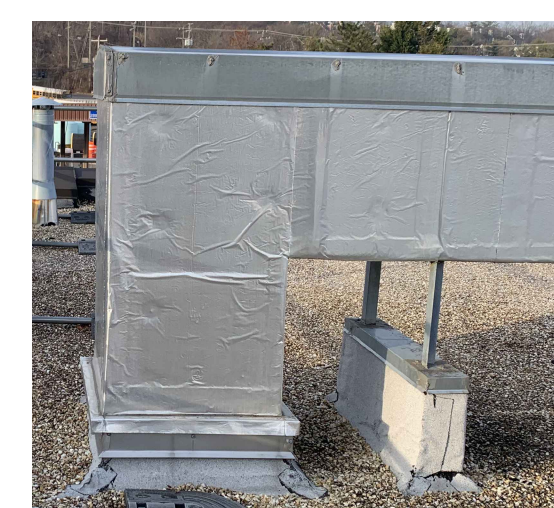
11 AD-102 NTS CURB AND DUCT SUPPORT (TYP)
