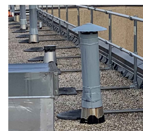
10 AD-102 NTS EXHAUST VENT PIPES (TYP)
