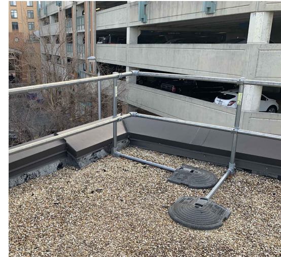
2 AD-102 NTS COPING AND GRAVITY RAILING (TYP)
