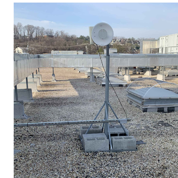
2 SATELLITE DISH ON BALLASTED STAND AD-104 NTS
