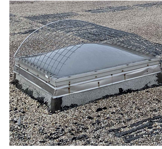
7 AD-102 NTS PROTECTION SCREEN AND SKYLIGHT (TYP)
