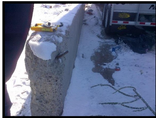
Figure 8 Barrier Wall Exposed Rebar
