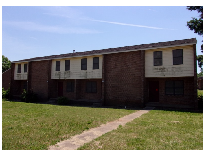
Photo 24 – Typical view of a 2-story, 4-unit building.
