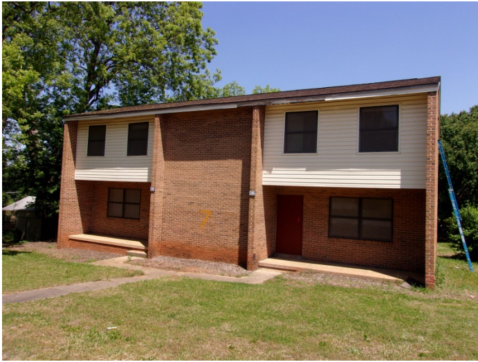
Photo 1 – Typical view of a 2-story duplex.
