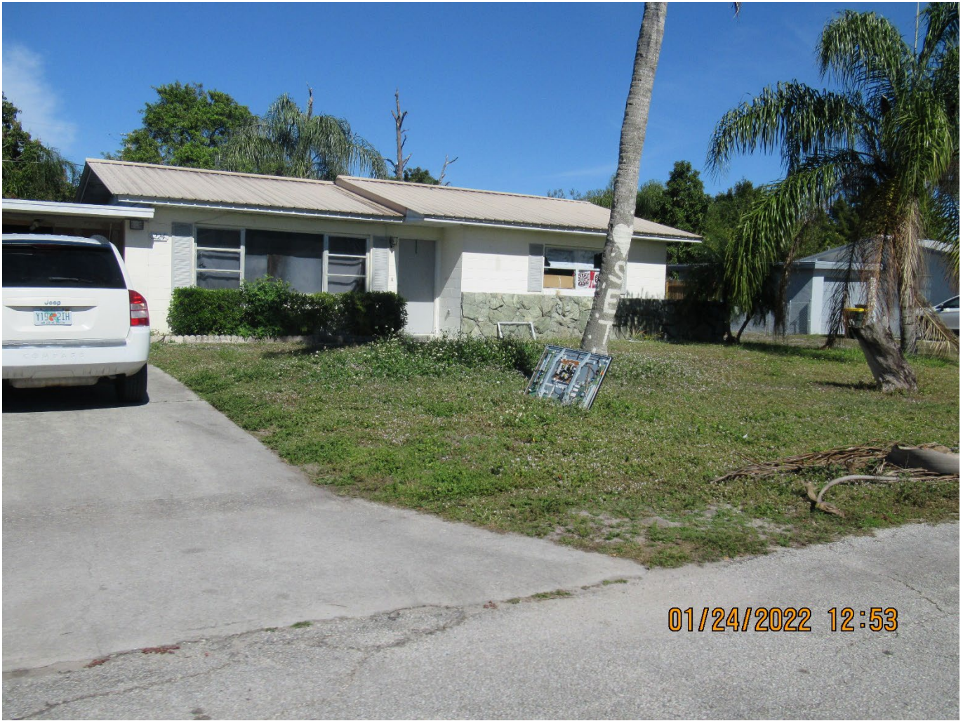
224 Sunnybrook Lane, Lake Placid, Florida, 33852 Parcel ID: C-22-37-30-030-00R0-0160
