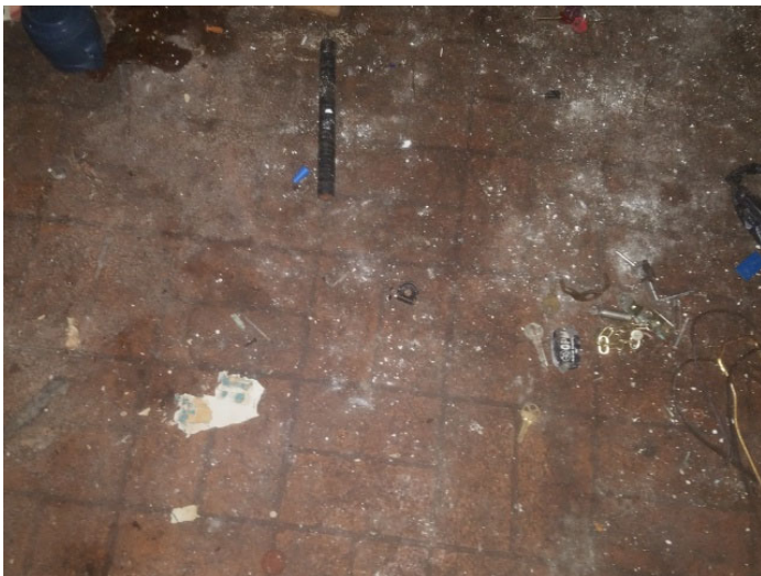
Photo 15 – Brown brick roll vinyl flooring in enclosed back porch
