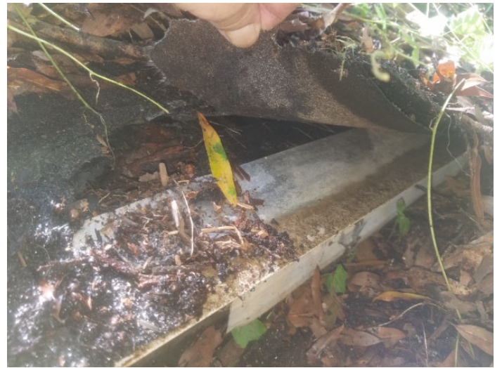
Photo 2 – One layer of shingle and felt
