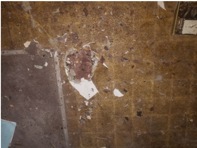
Photo 9 – Brown square vinyl flooring over gray spec roll vinyl over third layer with red bottom in middle room
