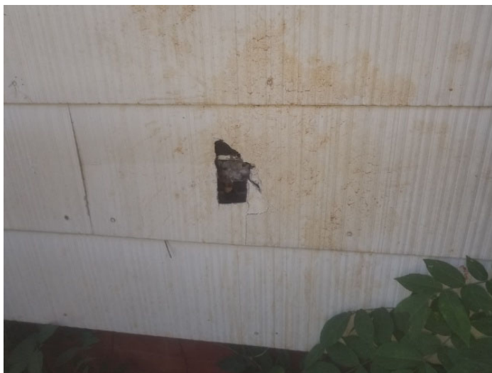
Photo 3 – White transite with felt
