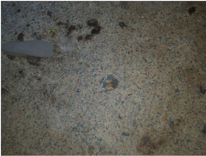
Photo 13 – Multi-color speckled roll vinyl flooring in left back room
