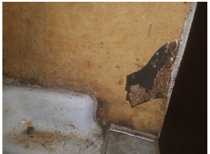
Photo 12 – Back splash located in the kitchen
