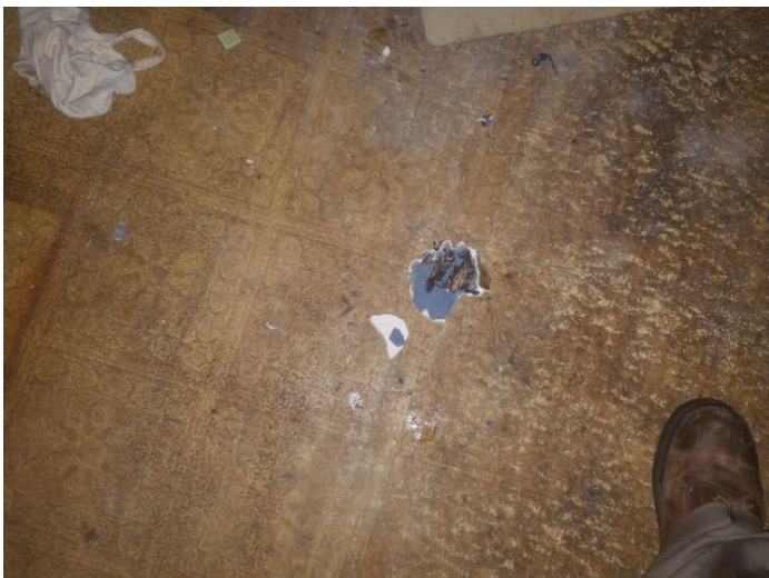
Photo 11 – Yellow large square pattern with blue felt in kitchen
