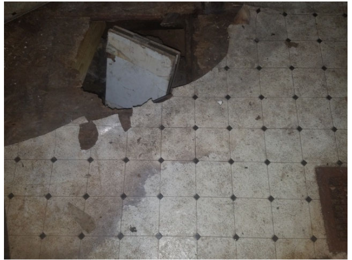
Photo 14 – White square with black diamond patterned roll vinyl in bathroom
