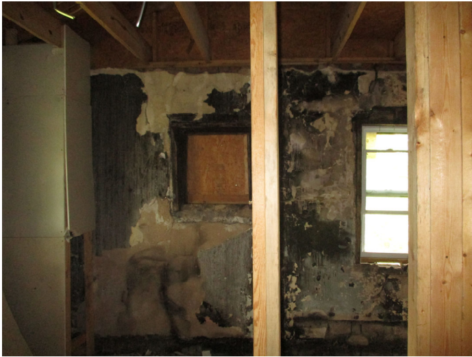
Photo 7 – Plaster with finish throughout walls.
