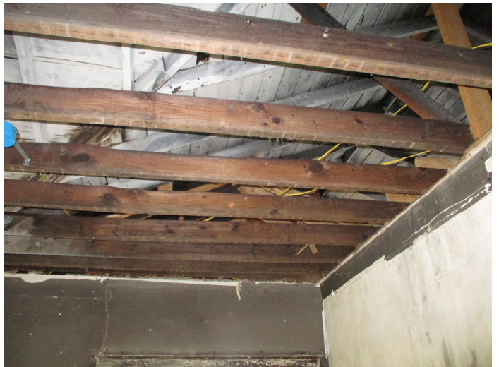
Photo 10 – Exposed ceiling joists.
