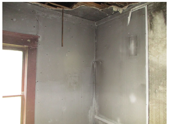
Photo 6 – Drywall and joint compound on walls scattered throughout.
