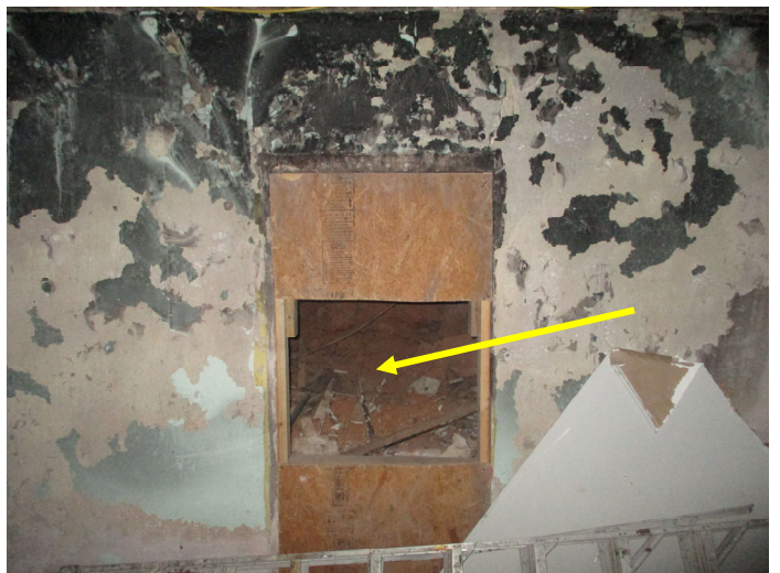
Photo 12 – Multiple types of layered vinyl flooring observed in porch crawlspace.
