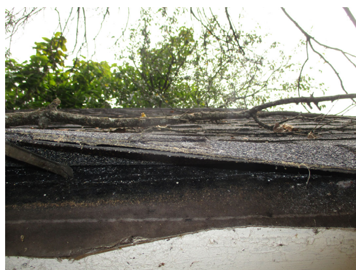
Photo 3 – One layer of shingle and one layer of felt.
