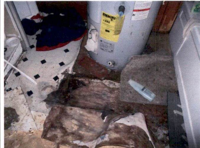
Photo 9 – Square and diamond pattern flooring over tan roll vinyl located in bathroom floor and shelves.
