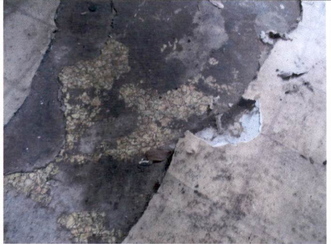
Photo 8 – Tan square roll vinyl flooring over tan/brown marble with green roll vinyl with adhesive in kitchen.
