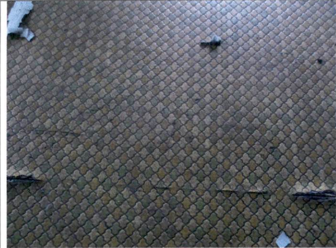
Photo 7 – Two layers of yellow roll vinyl with adhesive located in dining room and hallway.
