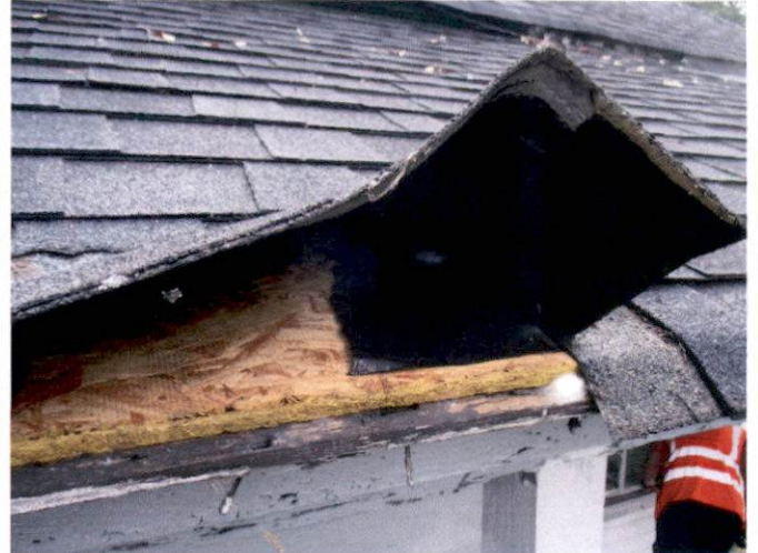
Photo 2 – One layer of shingle and felt
