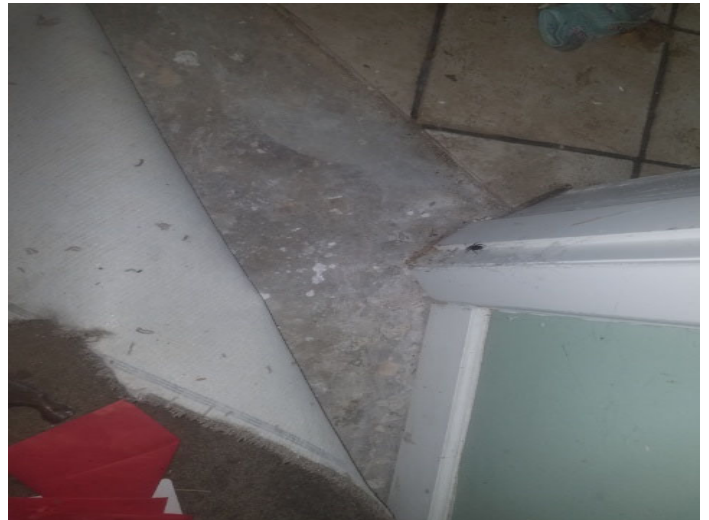
Photo 12 – Concrete floor under carpet.
