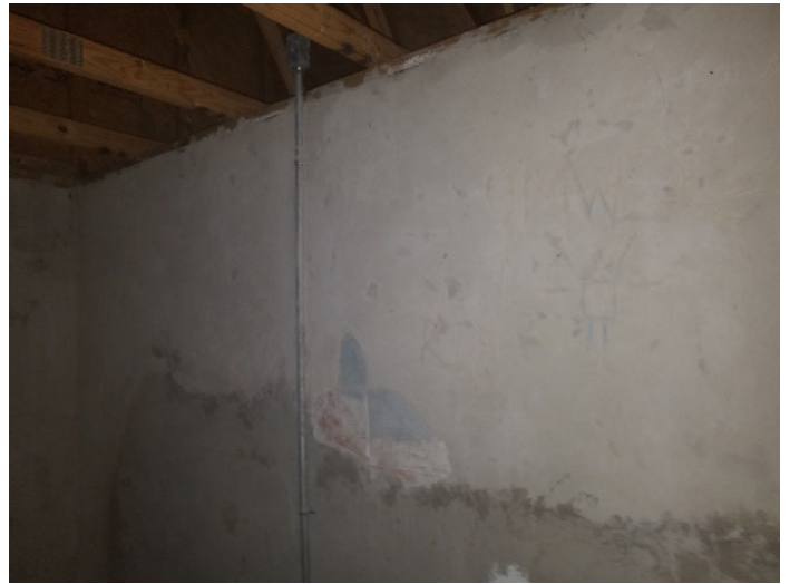
Photo 8 – Textured walls in unit 4 bedrooms.
