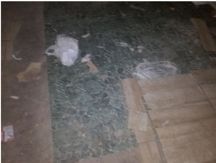
Photo 9 – Green marble floor tile located in unit 1 den and unit 4 hallway and kitchen.
