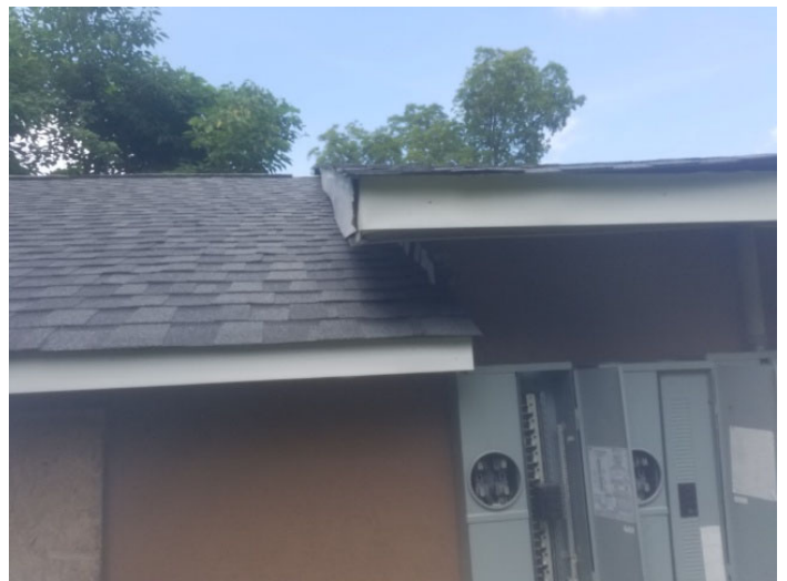
Photo 2 – Two sections of roofing material.
