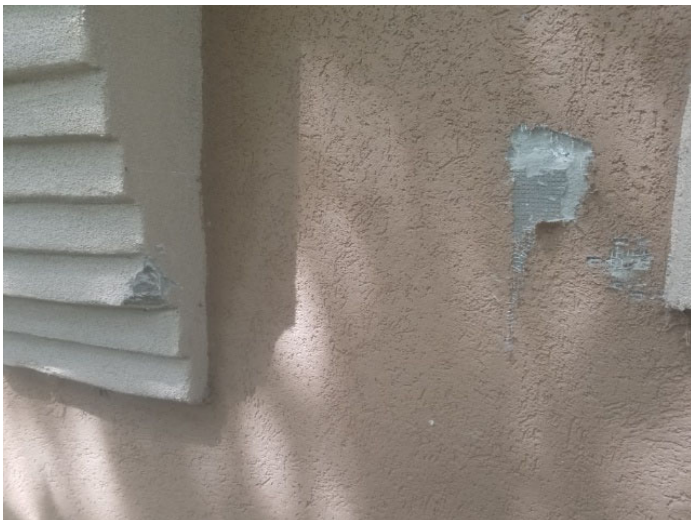
Photo 3 – Stucco and concrete exterior walls (EIFS).
