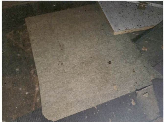
Photo 16 – Tan speckled roll vinyl with adhesive patch in kitchen.
