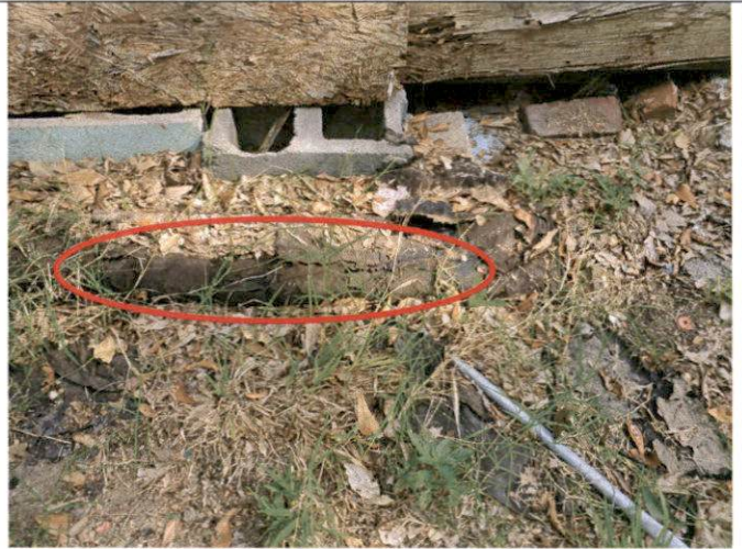
Photo 2 – Roll of black felt roofing material located on the ground near the house.
