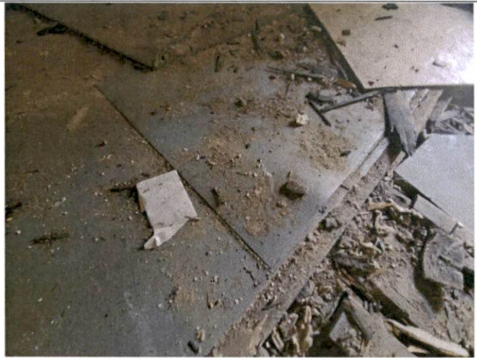
Photo 8 – Dark grey with specks roll vinyl with no mastic located in the living room.
