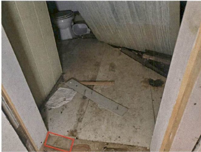
Photo 9 – Cream roll vinyl flooring located in bathroom.
