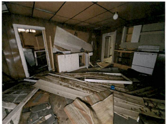
Photo 12 – Household debris throughout.
