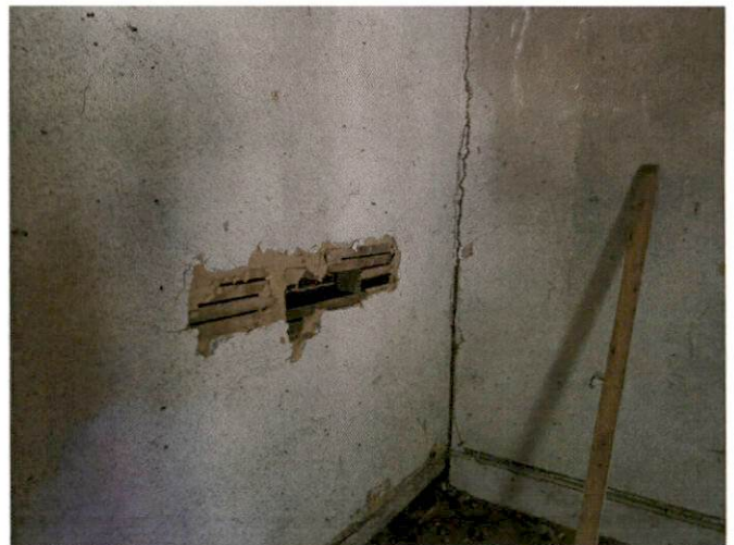
Photo 6 – Plaster, ceiling/wall texture and finish on ceiling and walls throughout.
