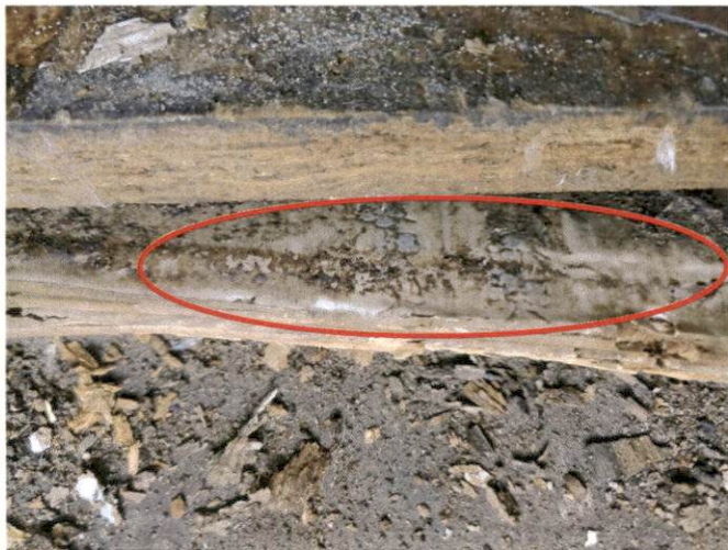
Photo 11 – White with blue flowers pattern roll vinyl flooring under wood flooring in the bathroom.
