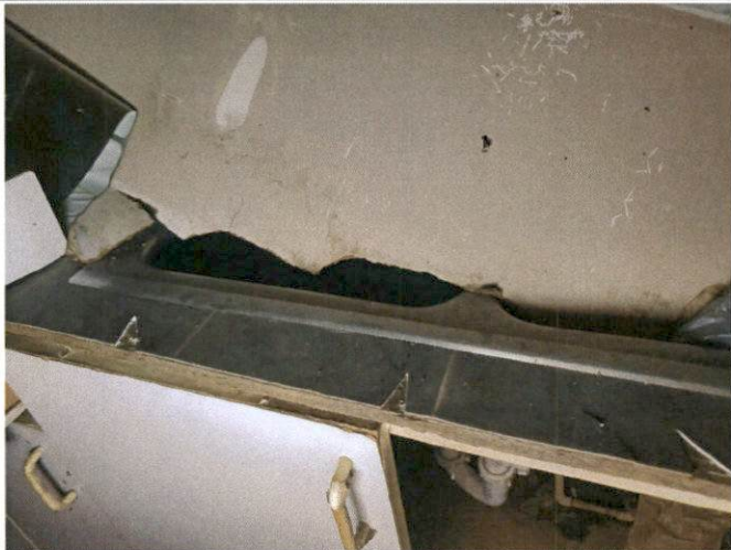
Photo 15 – Grey roll vinyl with adhesive located on kitchen counter.
