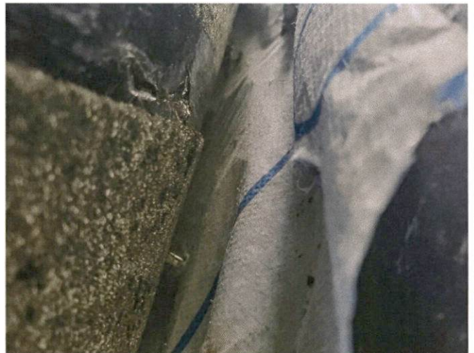
Photo 4 – Woven plastic material under shingles. Non - suspect ACM
