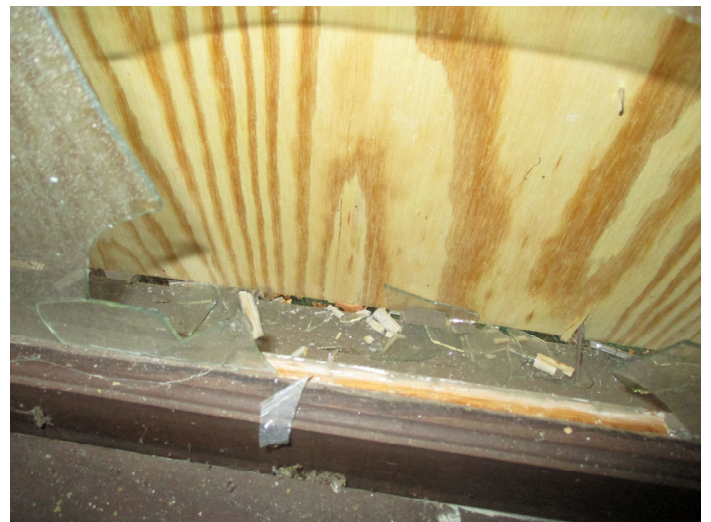
Photo 6 – Glazing found on wood windows
