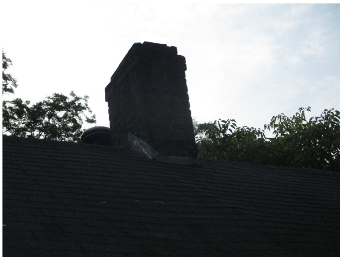
Photo 3 – Chimney tar assumed asbestos containing material.
