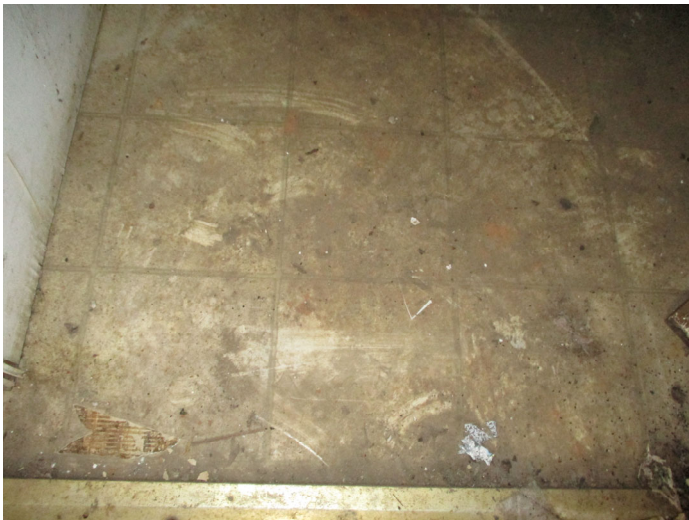
Photo 15 – Plain tan square roll vinyl floor with no adhesive located in the bathroom.
