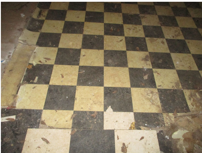
Photo 11 – Black and white roll vinyl floor & mastic located in the kitchen
