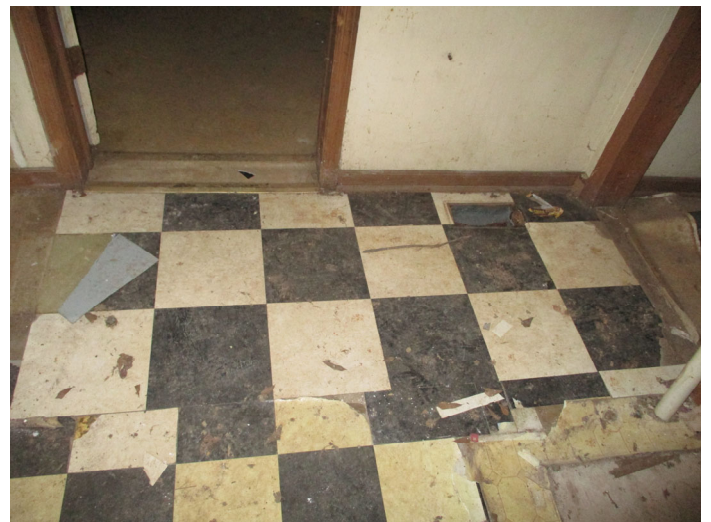
Photo 12 – Back and white 12"x12" self-stick floor tiles located in the kitchen
