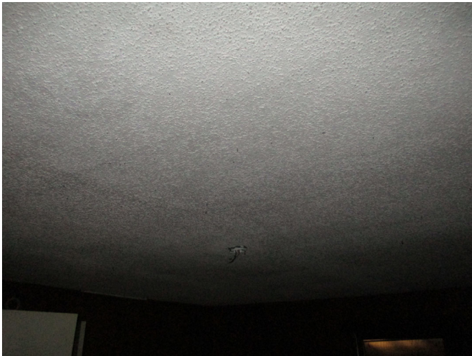
Photo 7 – Ceiling texture throughout.
