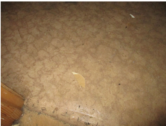
Photo 17 – Brown pebble roll vinyl floor & mastic in the back left room closet.
