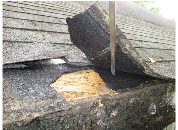
Photo 2 – One layer of shingle and felt
