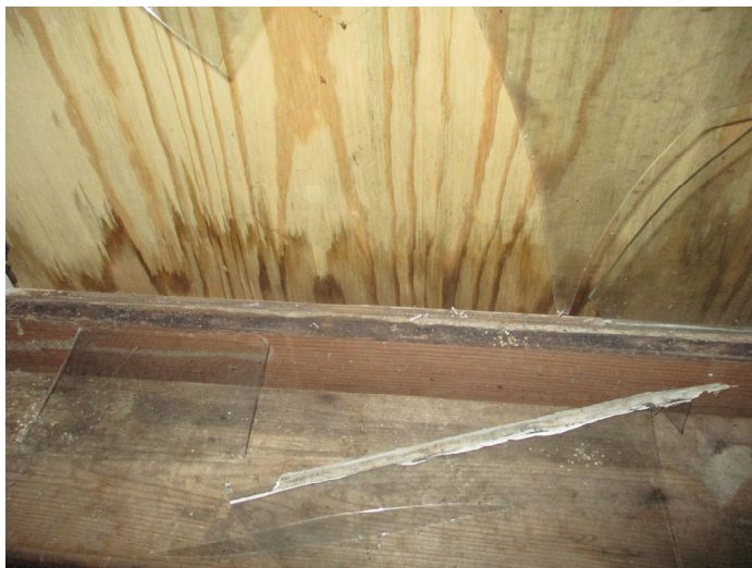
Photo 5 – Glazing found on wood windows
