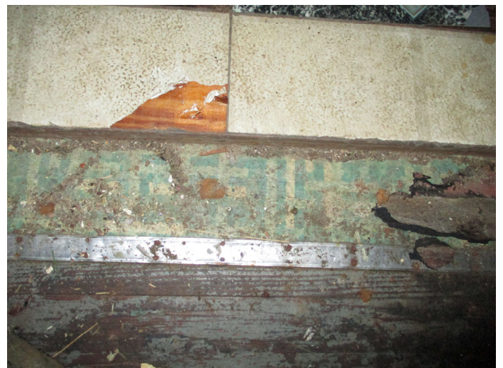
Photo 16 – Tan and blue vinyl flooring under thin wood floor in bathroom.
