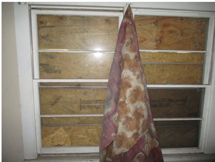
Photo 5 – Typical view of wood windows.
