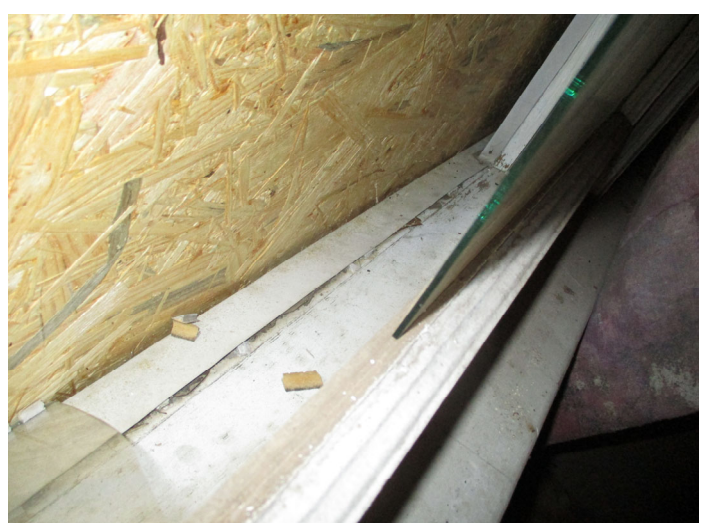
Photo 4 – Glazing on wood windows.
