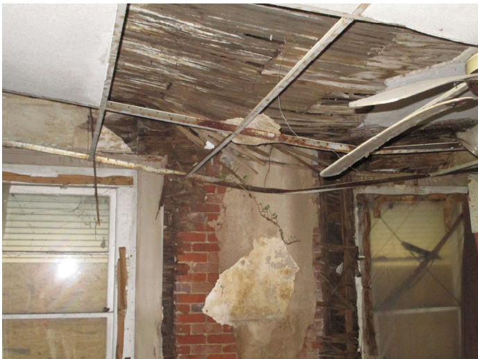
Photo 9 – Plaster with finish and drywall walls throughout.
