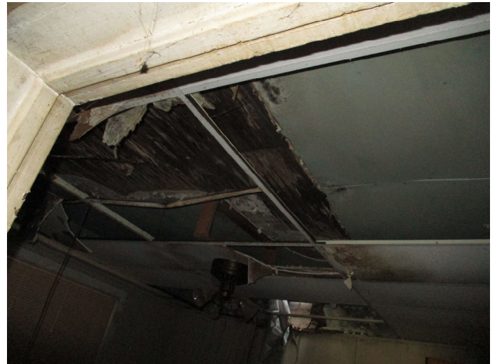
Photo 14 – Wood ceiling above ceiling grid and plaster.
