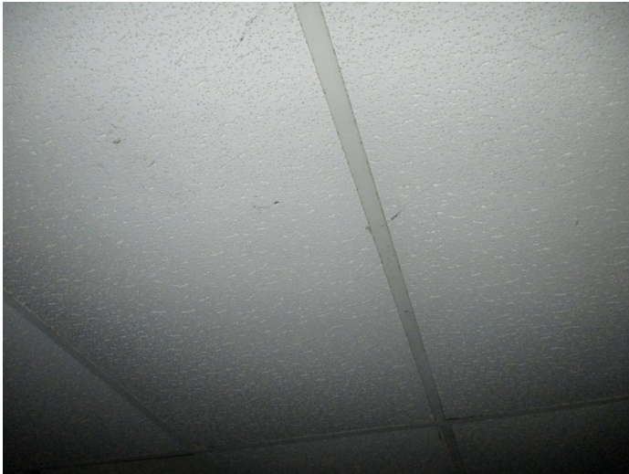
Photo 7 – 2'x4' worm hole pattern ceiling tile sporadically throughout.
