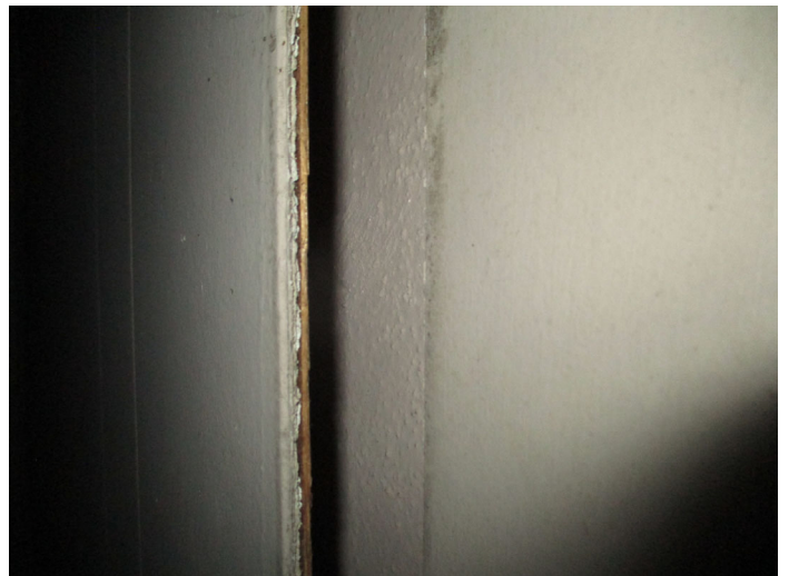
Photo 10 – Wood paneling over plaster walls
