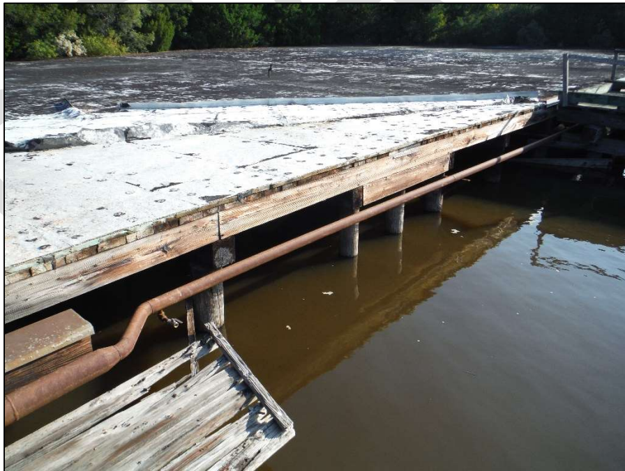
Photograph A 6 – South Face of North Section Looking Northeast
