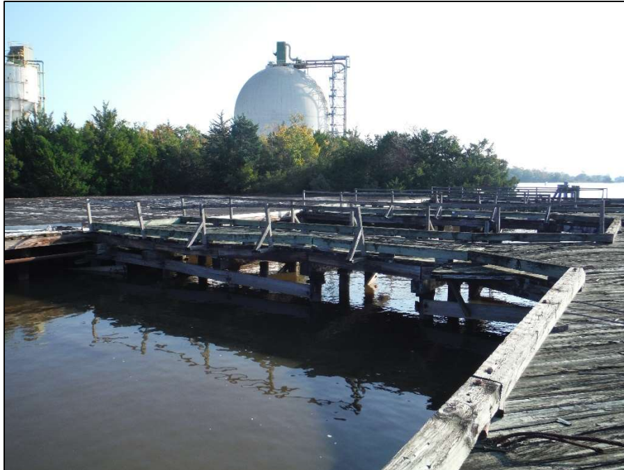
Photograph A 5 – Typical Approach Pier Looking Northeast
