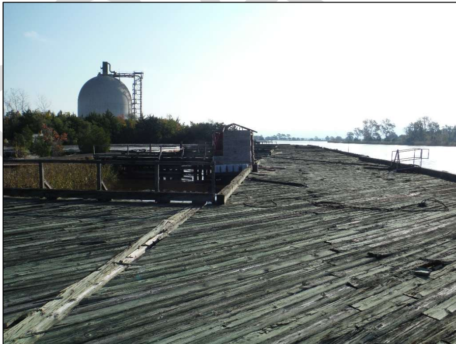
Photograph A 4 – Overall Dock Looking East
