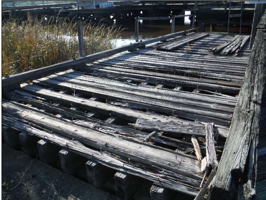
Photograph A 3 – Overall Dock Looking South
