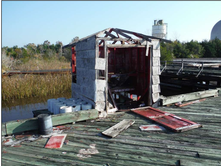
Photograph A 9 – Storage Shed on South Edge Looking Northeast
