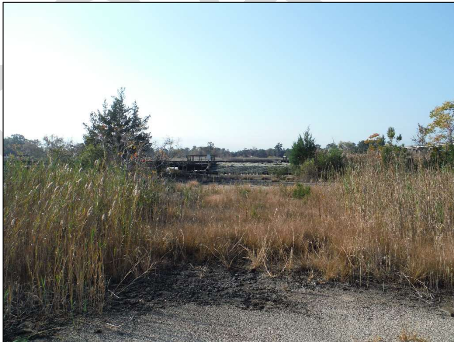
Photograph A 2 – Overall Dock Looking South
