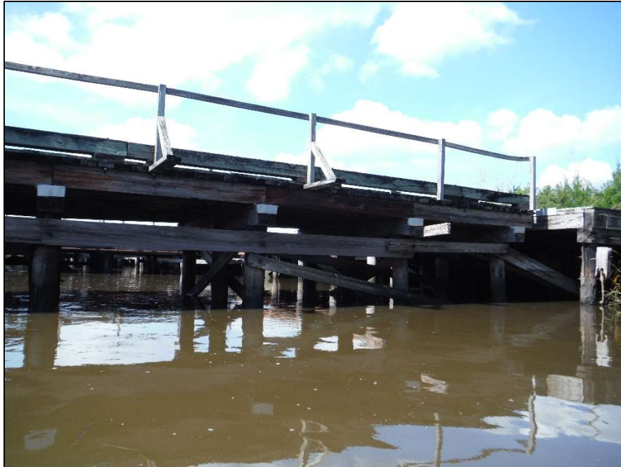
Photograph A 11 – Typical Railing
