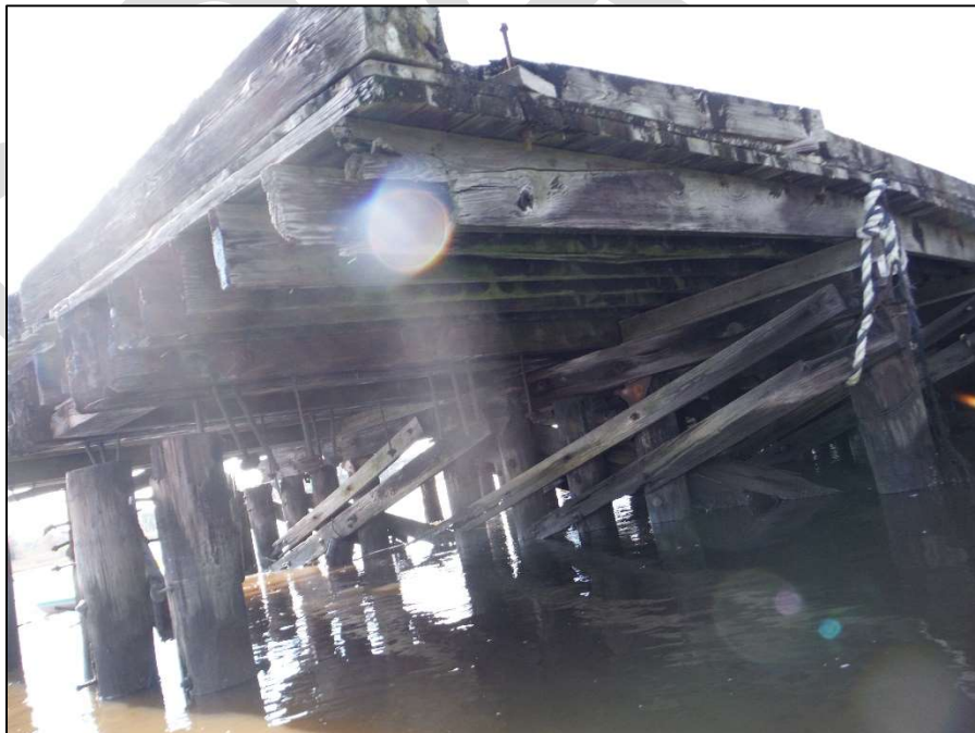
Photograph A 12 – Typical Underside of Deck
