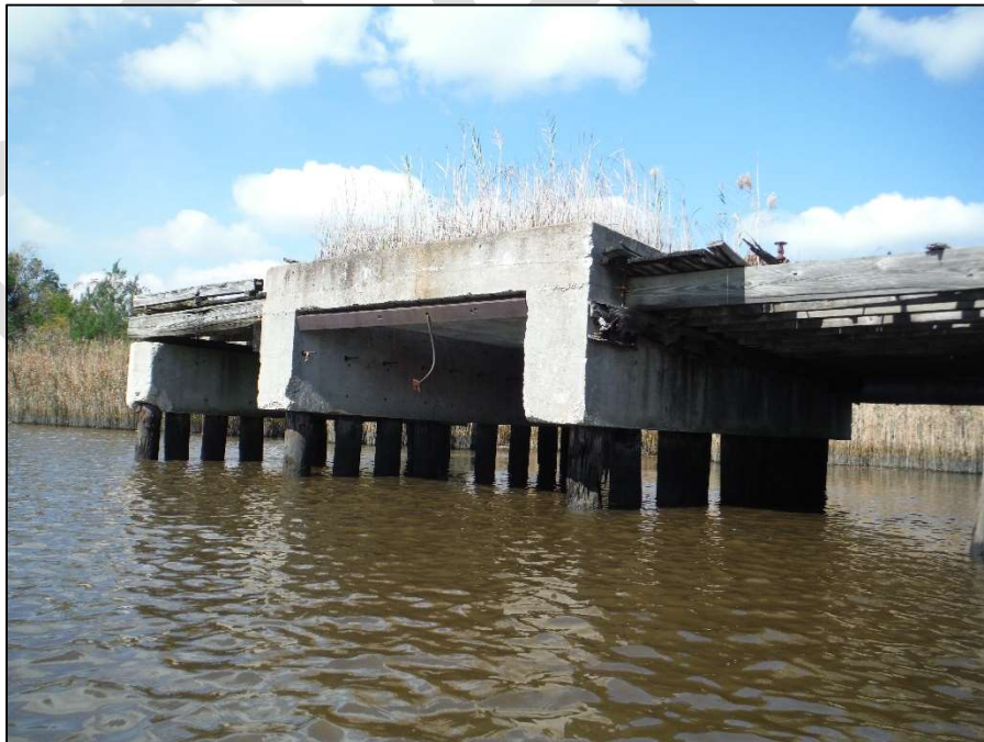
Photograph A 10 – West End of South Fascia Looking Northwest
