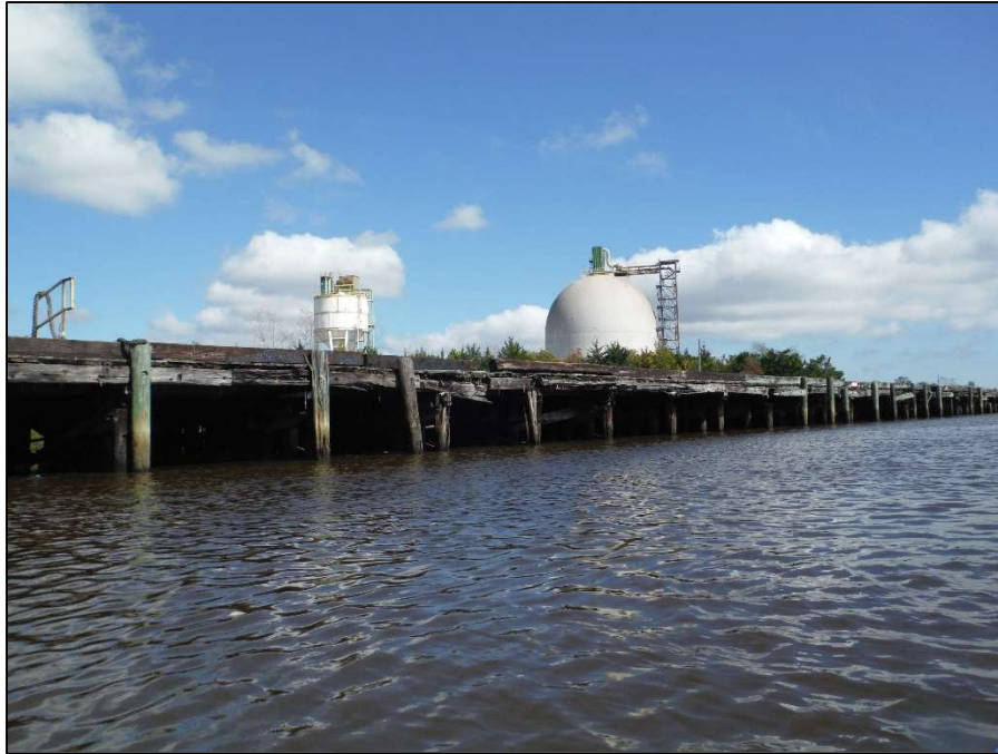
Photograph A 1 – Overall Abandoned Timber Dock Looking Northeast (South Fascia Shown)
