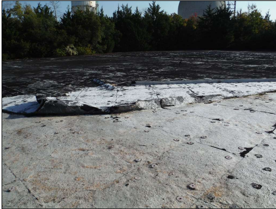
Photograph A 7 – Typical Deck at North Dock Section Looking Northeast
