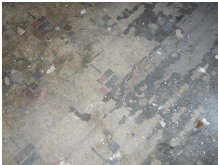
Photo 10 – Residual vinyl floor in kitchen.
