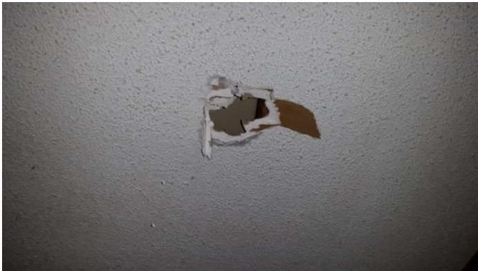
Photo 3 – Ceiling texture over drywall.
