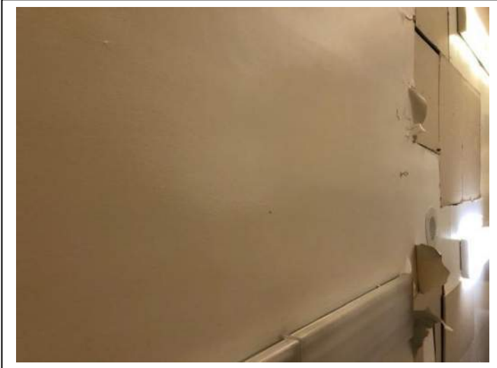
Photo #41 Material: Smooth Plaster Sample Result: No Asbestos Detected
