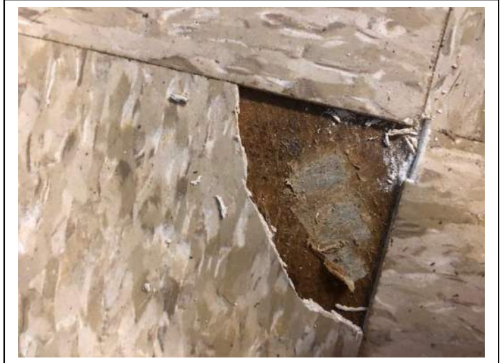
Photo #42 Material: Tan Floor Tile Mastic Sample Result: No Asbestos Detected
