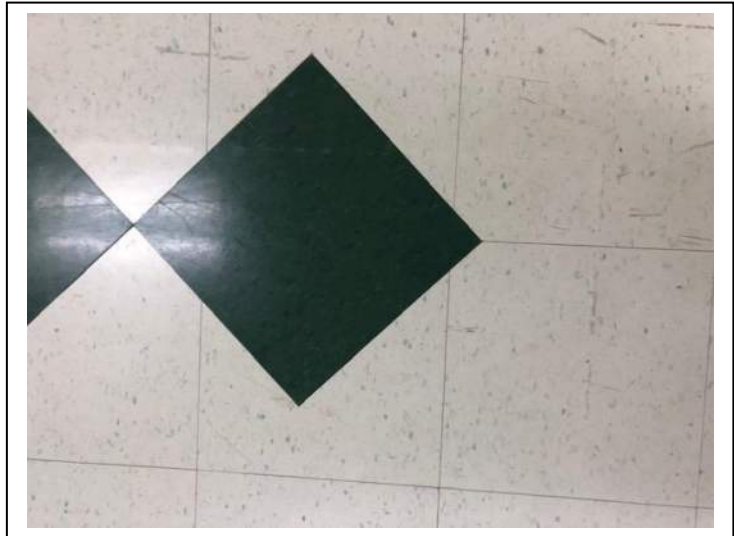
Photo #54 Material: 12"x12" Green Mottled Floor Tile Sample Result: No Asbestos Detected
