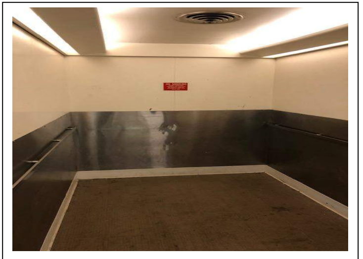
Photo #84 Material: Elevator Cab Insulation Sample Result: Assumed ACM
