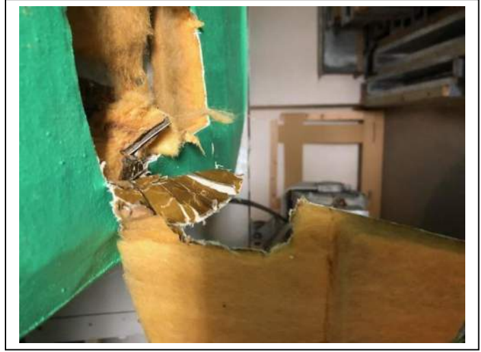
Photo #18 Material: Green Canvas Duct Sample Result: No Asbestos Detected
