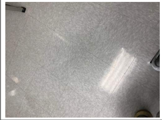
Photo #29 Material: 12"x12" Gray Mottled Floor Tile Sample Result: No Asbestos Detected
