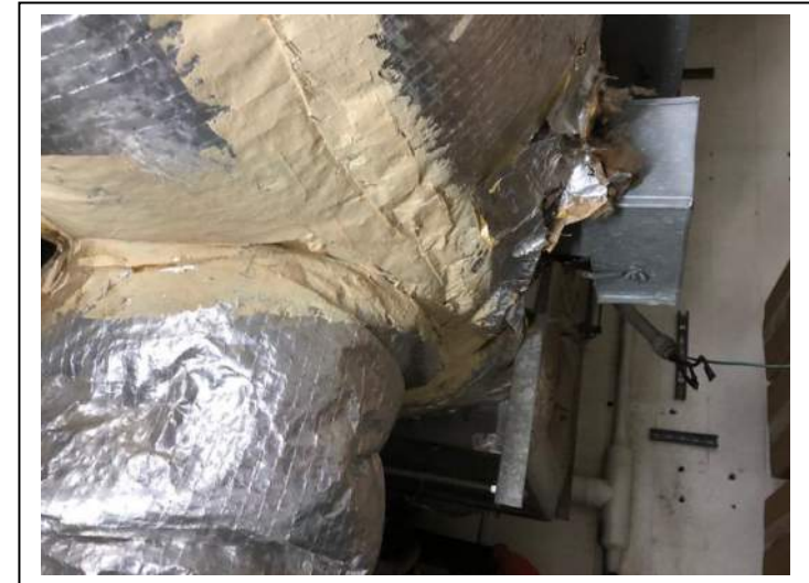
Photo #48 Material: Tan Duct Seam Sealant on foil Sample Result: No Asbestos Detected
