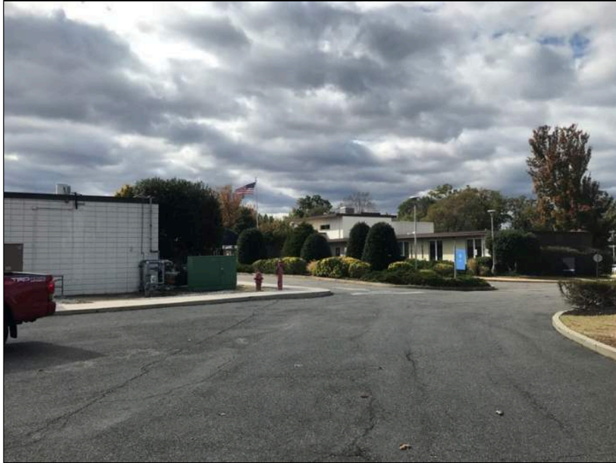
1 - View of the Northern One-Story and Two-Story Sections of the Building.
