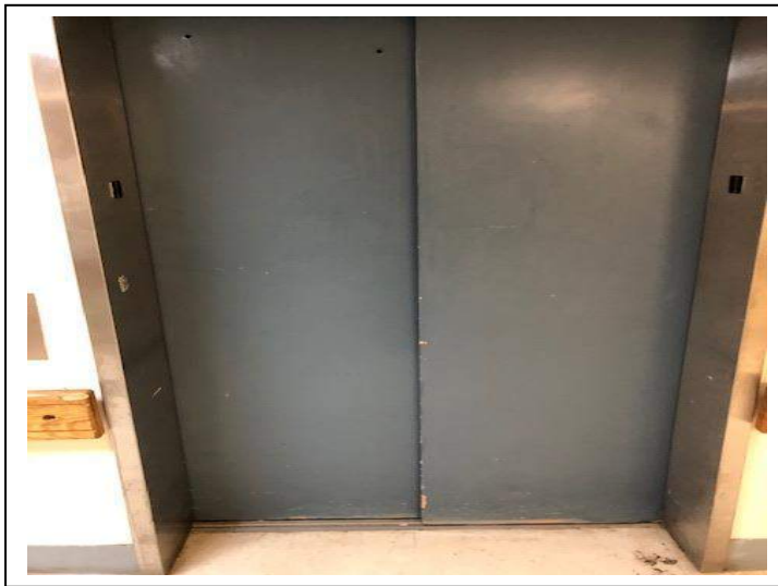
Photo #83 Material: Elevator Door Insulation Sample Result: Assumed ACM
