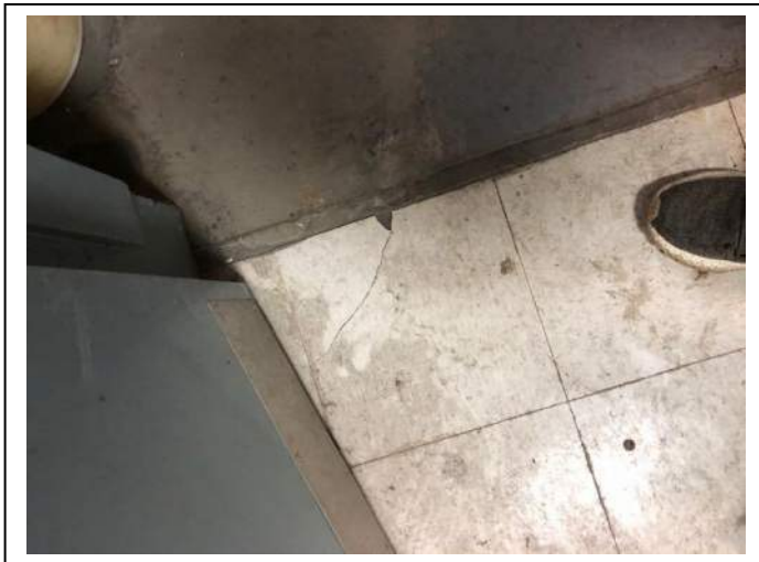
Photo #35 Material: 12"x12" White Floor Tile Sample Result: No Asbestos Detected
