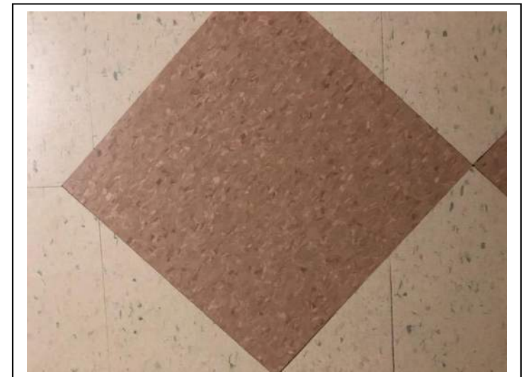
Photo #44 Material: 12"x12" Pink Mottled Floor Tile Sample Result: No Asbestos Detected
