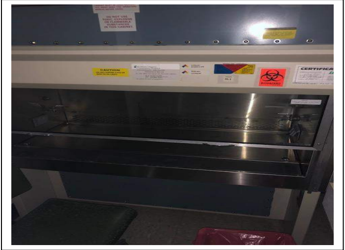
Photo #6 Material: Transite Fume Hood Sample Result: Not Sampled
