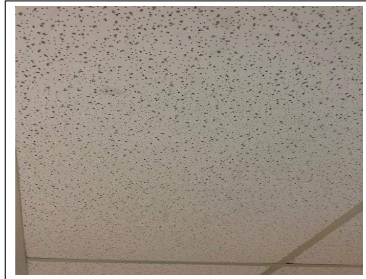
Photo #63 Material: Cratered Pinhole Ceiling Tile Sample Result: No Asbestos Detected
