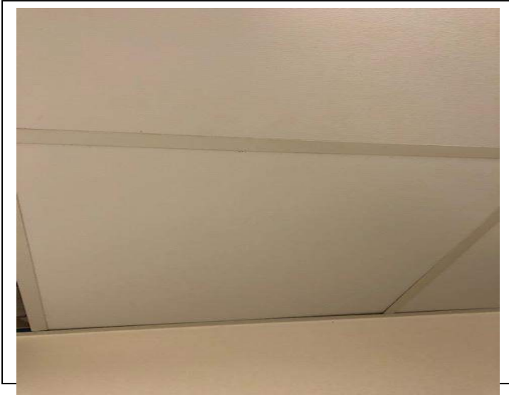
Photo #61 Material: Smooth Pinhole Ceiling Tile Sample Result: No Asbestos Detected
