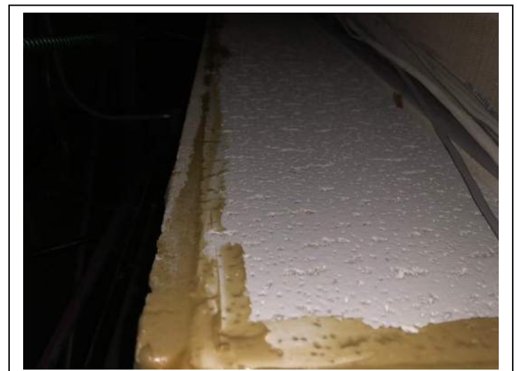
Photo #80 Material: Tan Light Mastic Sample Result: No Asbestos Detected
