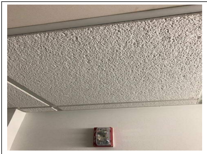
Photo #67 Material: Textured Ceiling Tile Sample Result: No Asbestos Detected
