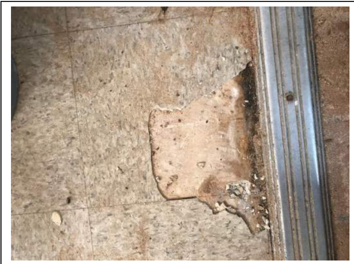
Photo #79 Material: 12"x12" Pink Floor Tile Sample Result: No Asbestos Detected
