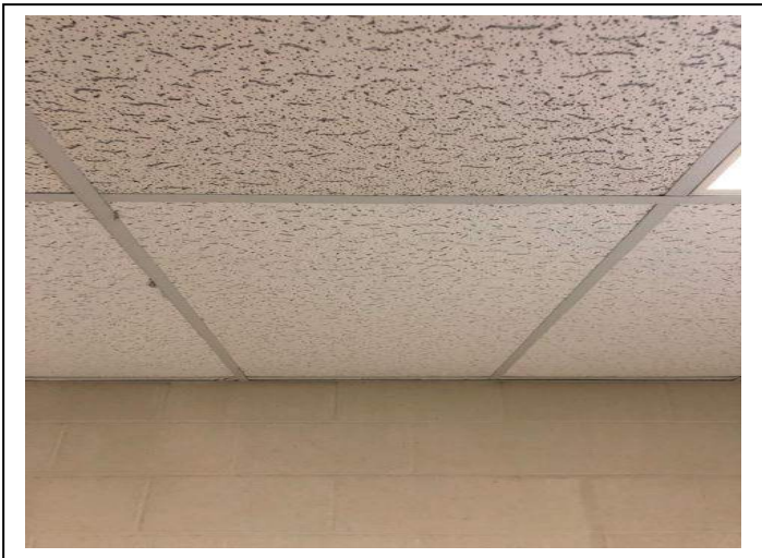
Photo #3 Material: Fissure Pinhole Ceiling Tile Sample Result: No Asbestos Detected
