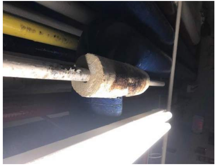
Photo #72 Material: End Cap Sealant (Old) Sample Result: No Asbestos Detected
