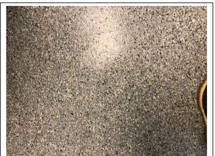
Photo #76 Material: 12"x12" Blue Multi-Speck Floor Tile Sample Result: No Asbestos Detected
