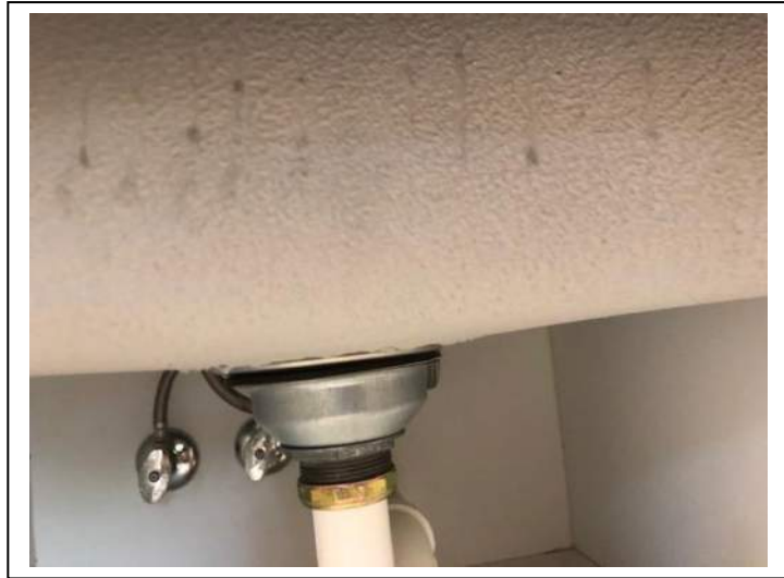
Photo #66 Material: Sink Trap Sample Result: Potential Mercury
