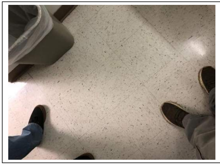
Photo #68 Material: 12"x12" White with Black Specks Sample Result: No Asbestos Detected
