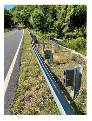
Remove & replace <u>+</u>75 damaged W-Beam system. Reset 1 additional post. Replace an additional 4 offset blocks at various locations.
